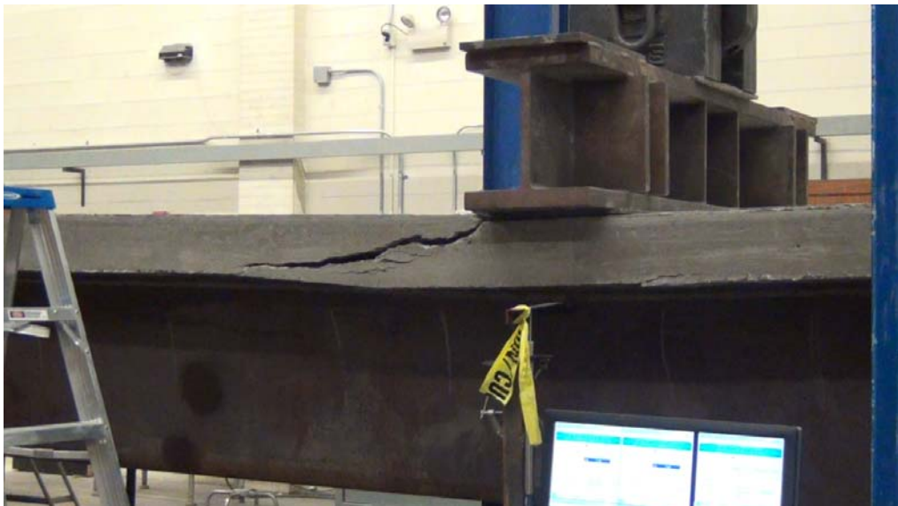
Figure 4.16: Typical Failure Mode for Composite Specimens
