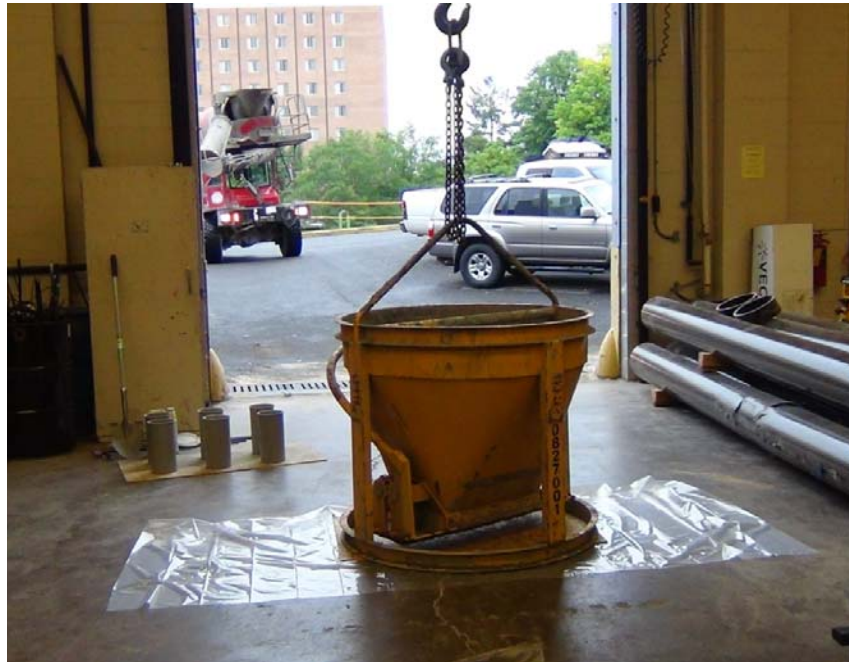
Figure 4.12: Concrete Bucket Used for Deck Placement
