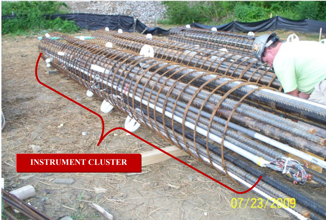
Figure 3-28 Rebar cage after installation of all gages.
