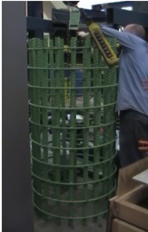
Figure 3-8 Assembled rebar cage prior to trial caisson testing.
