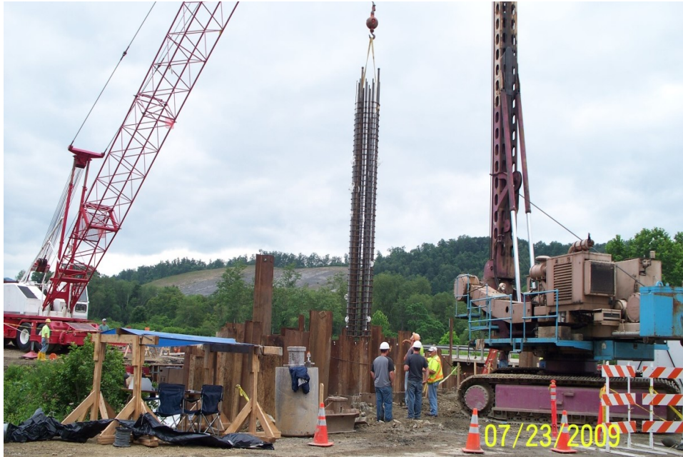
Figure 3-29 Placement of rebar cage for use in Stalnaker Run caisson, Abutment 2.
