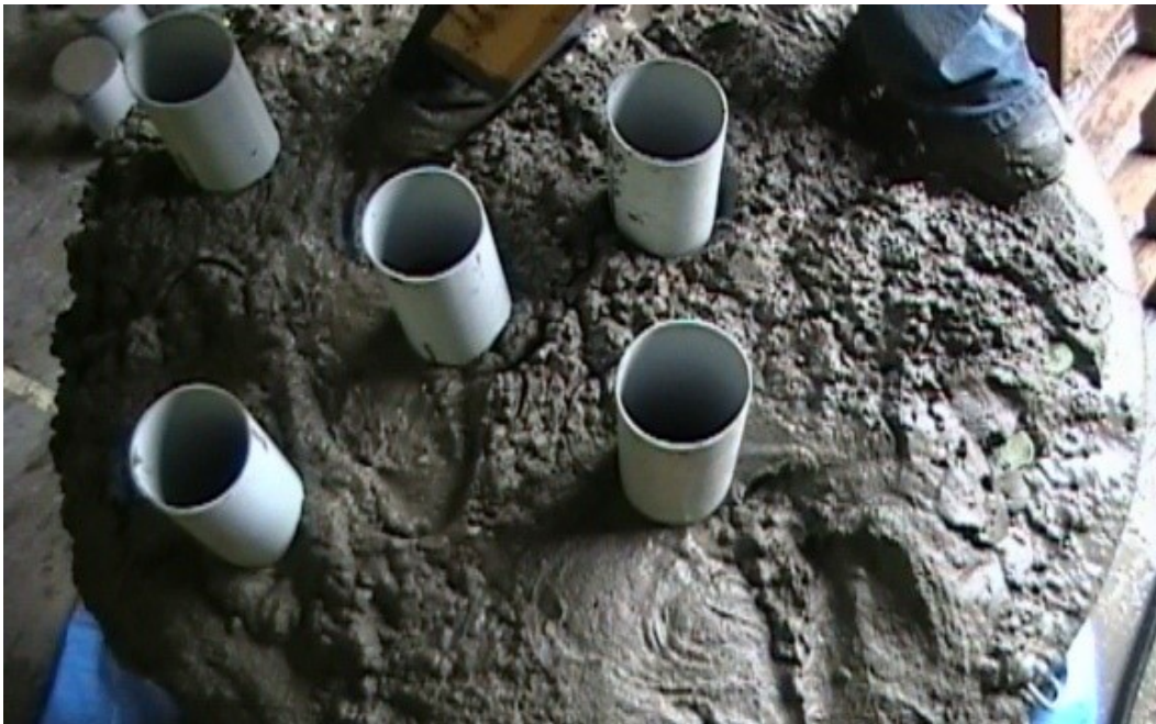
Figure 3-10 Locations of trial caisson fresh core tubes, as placed.
