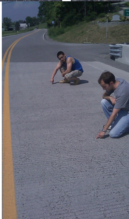
Figure 5-17 Observed longitudinal cracking of Stalnaker Run Bridge Deck. (a) Crack initiating at Abutment #1, (b) crack initiating at Abutment #2, and (c) crack present near midspan.
