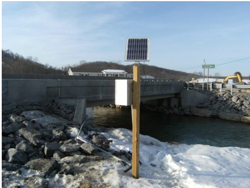
Figure 5-8 Long-term monitoring station adjacent to the Stalnaker Run Bridge. Upstream location, south bank.
