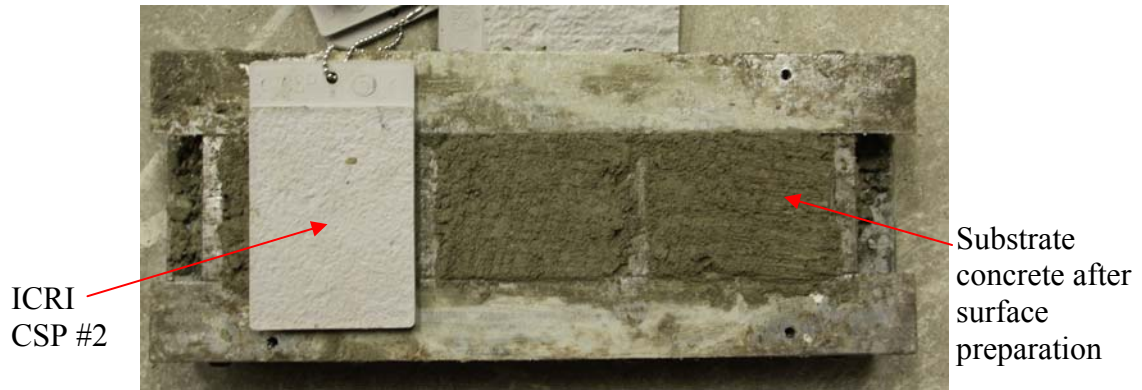
Fig. 3.9 Substrate surface preparation
