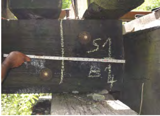
Figure 42 - Span 1 Stringer 1 end rot over Bent 1 (left) and Span 1 Stringers 1 & 2 end rot over Bent 1(right).
