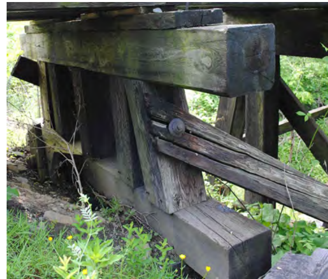
Tower Brace 1 West
