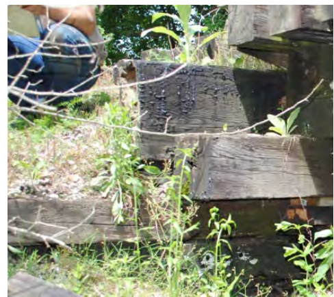
Figure 41 - South Backwall and South West Wingwall heart rot (left). North Backwall West End heart rot (right)
