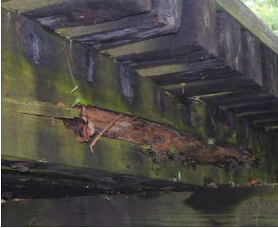
Figure 47 - Span 3 & 4 Stringer 8 highly rotted (left) and Span 1 Stringer 1 East face fruiting bodies (right).
