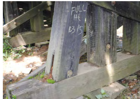
Figure 43 - Bent 3 Corbel 2 rot (left) and Bent 3 Post 5 heart rot (right).
