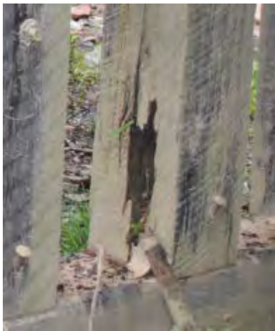
Figure 48 - Bent 5 Post 3 heart rot (left) and Bent 3 Sill end rot (right).
