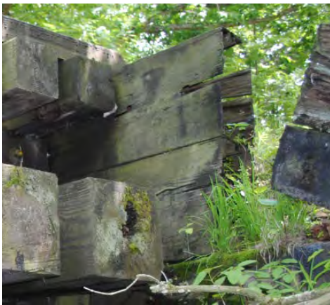
Figure 41 - South Backwall and South West Wingwall heart rot (left). North Backwall West End heart rot (right)
