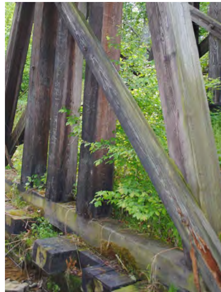
Bent 6 - North Sway Brace
