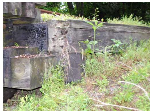
Figure 46 - South Retaining Wall & West Wingwall (left) and North East Wingwall heart rot (right).
