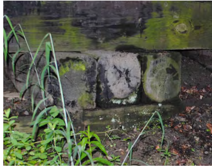
Bent 1 - Blocks 5 & 6 Softening
