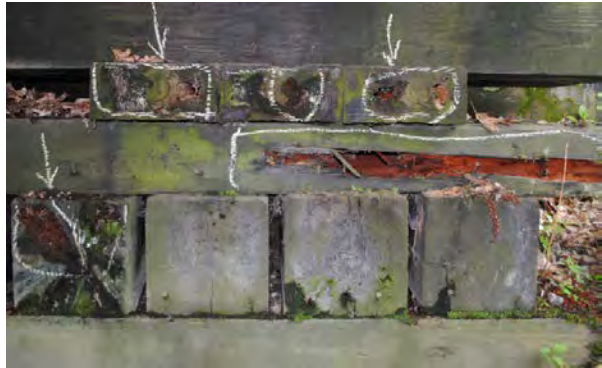
Figure 44 - Bent 2 Post 1 heart rot (left) and Bent 4 Blocks & Sills rot (right).
