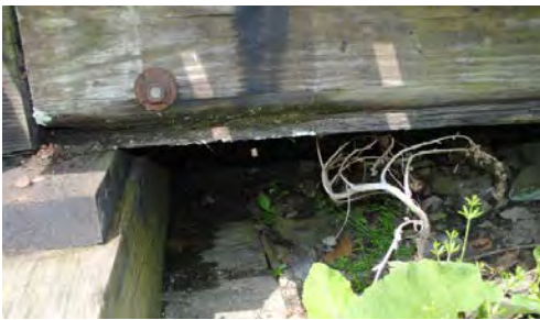
Figure 36 – Rot Span 1 Stringer 1 over Bent 2 (left) and Span 3 Stringer 2 (second stringer from the top down) rotting (right).
