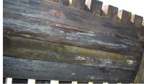
Figure 36 – Rot Span 1 Stringer 1 over Bent 2 (left) and Span 3 Stringer 2 (second stringer from the top down) rotting (right).
