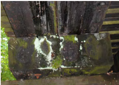
Figure 43 - Bent 3 Corbel 2 rot (left) and Bent 3 Post 5 heart rot (right).
