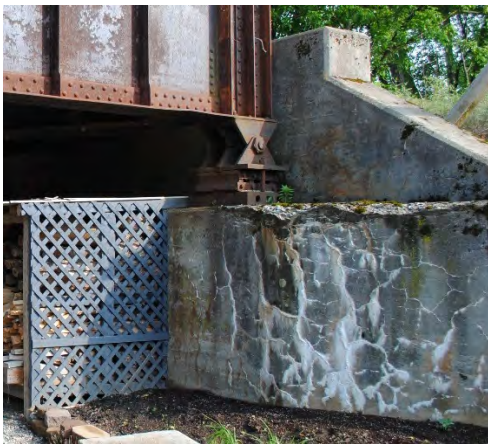
Figure 51 - Map cracking in north abutment (left) and pier (right)
