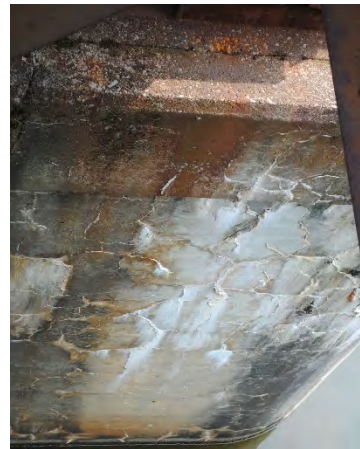
Figure 51 - Map cracking in north abutment (left) and pier (right)
