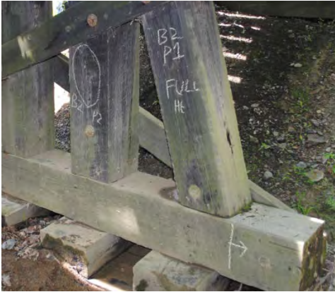
Figure 44 - Bent 2 Post 1 heart rot (left) and Bent 4 Blocks & Sills rot (right).
