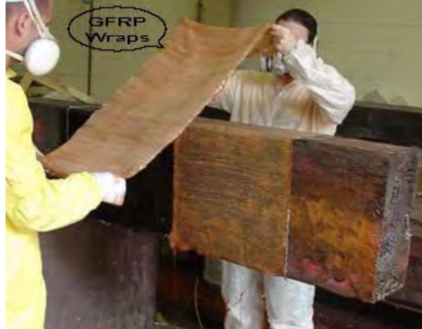
Figure 1 - Timber Stringer Rehabilitation using GFRP (Abhari, 2007)
