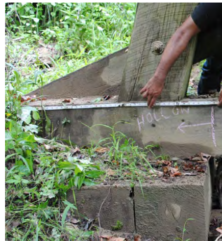
Figure 48 - Bent 5 Post 3 heart rot (left) and Bent 3 Sill end rot (right).
