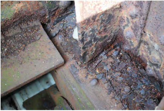
Figure 50 - Corrosion in angle of girder (left) and corrosion in gusset plate & web stiffeners (right)
