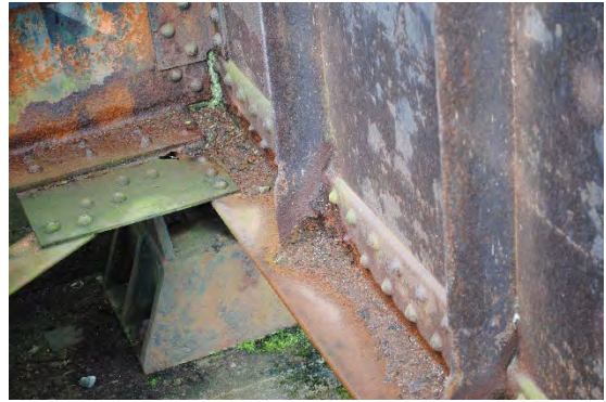
Figure 50 - Corrosion in angle of girder (left) and corrosion in gusset plate & web stiffeners (right)
