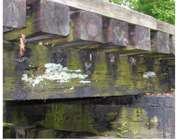
Figure 47 - Span 3 & 4 Stringer 8 highly rotted (left) and Span 1 Stringer 1 East face fruiting bodies (right).
