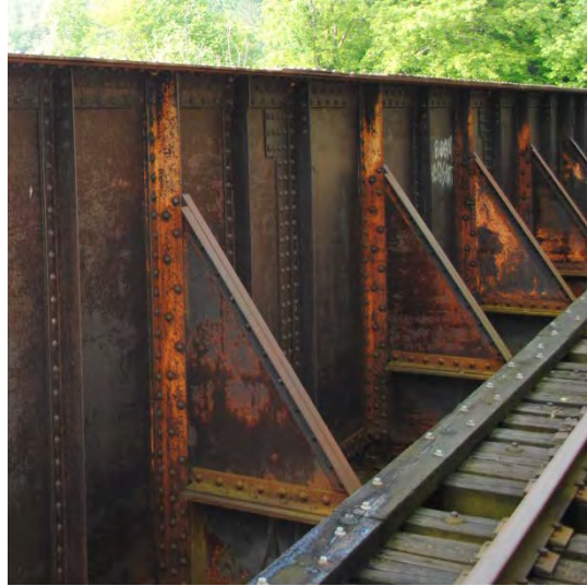
Figure 62 - Triangular Stiffeners on Floor Beam Top Flanges (Bridge 1.4)
