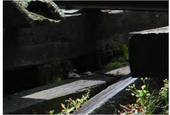
Figure 42 - Span 1 Stringer 1 end rot over Bent 1 (left) and Span 1 Stringers 1 & 2 end rot over Bent 1(right).
