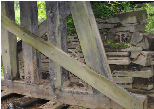
Figure 46 - South Retaining Wall & West Wingwall (left) and North East Wingwall heart rot (right).
