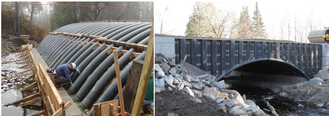
Figure 1.7: Civil engineering application: Inflatable Composite Bridge [13].
