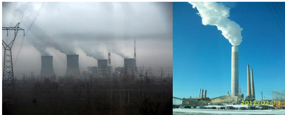
Figure 7.6 No air pollution control devices (left), with air pollution control devices(right) (Miller, 2011)
