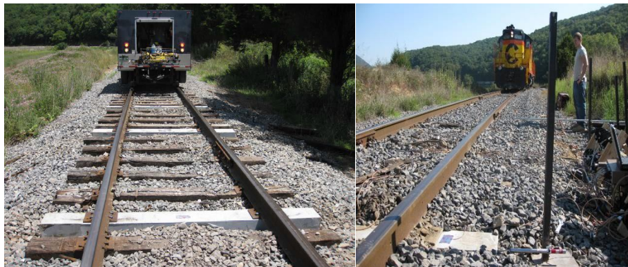
Figure 6.3 Field Testing of Recycled GFRP Composite Railroad Ties (256 Kips) on SBVR Line in Moorefield, WV (Chada, 2012)
