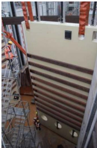
Figure 2.12 Lock Doors Wilhelminakanaal Tilburg, (The Netherlands, 2016)
