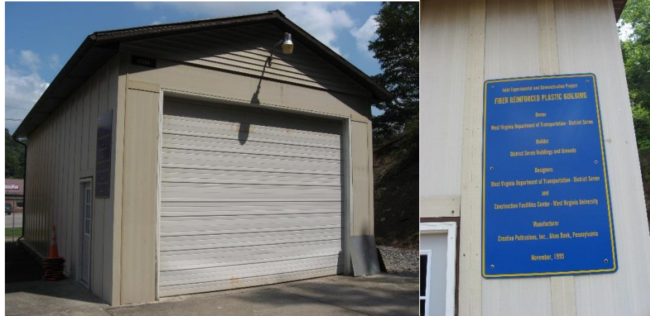
Figure 7.16 Multi-purpose FRP Building, Weston, WV, Nov. 1995 (photos taken on Aug 27, 2009)
