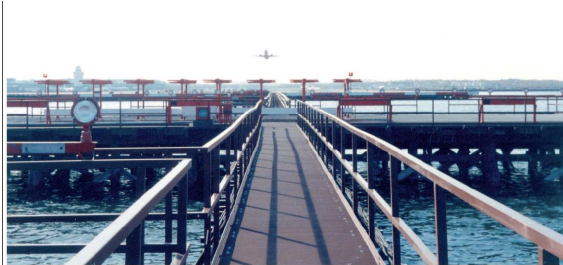
Figure 8.28 DURADEK platforms and catwalks
