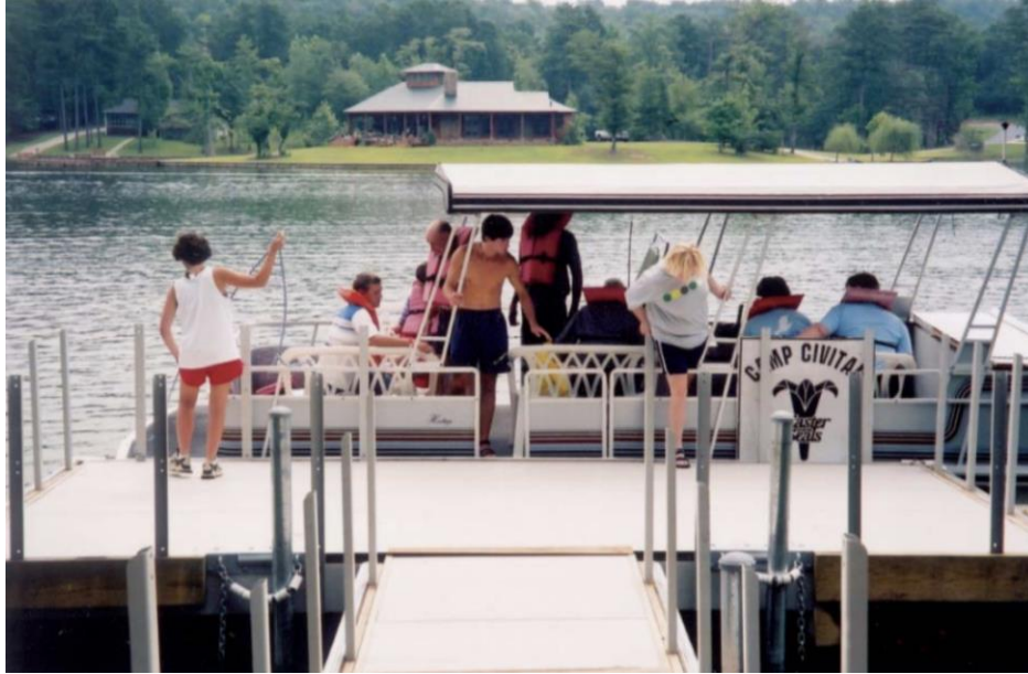
Figure 8.8.34 Strongwell's SAFPLANK® fiberglass plank system for the pier's deck
