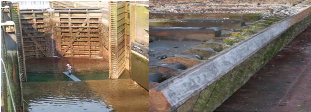
Figure 8.1 Miter Gate (left); Miter Block (right)
