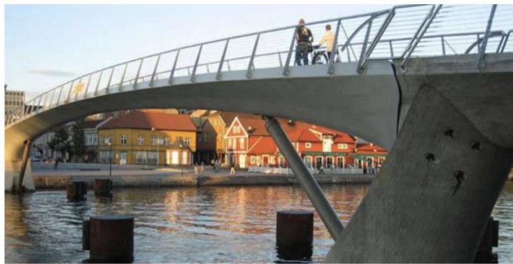
Figure 2.15 Bridge Fredrikstad, 60 m span pedestrian bridge, (Norway, 2018)
