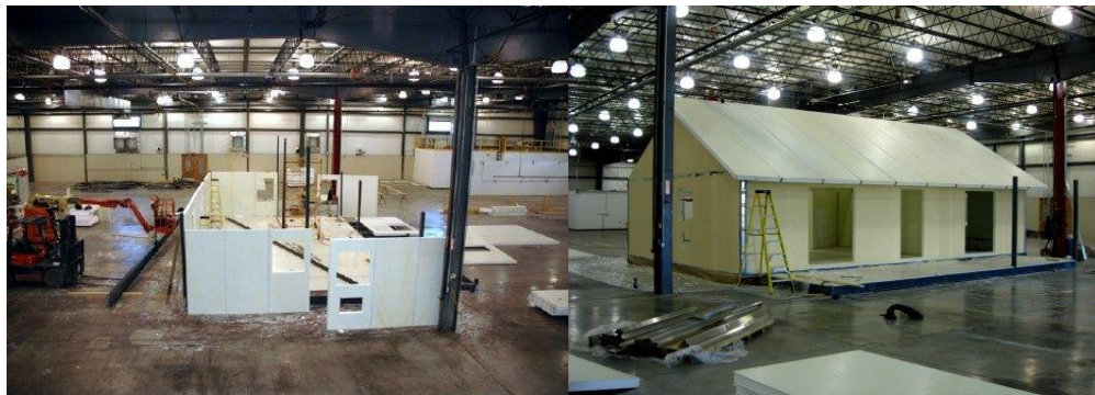
Figure 7.17 FRP Composite House at Bedford Reinforced Plastics Inc. Facility (2008) (courtesy of Bedford Reinforced Plastics Inc)
