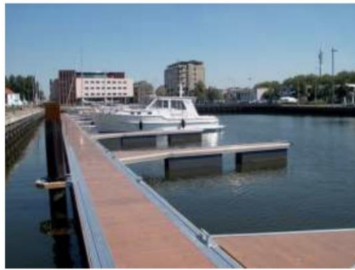
Figure 2.21 Jetty and catwalks
