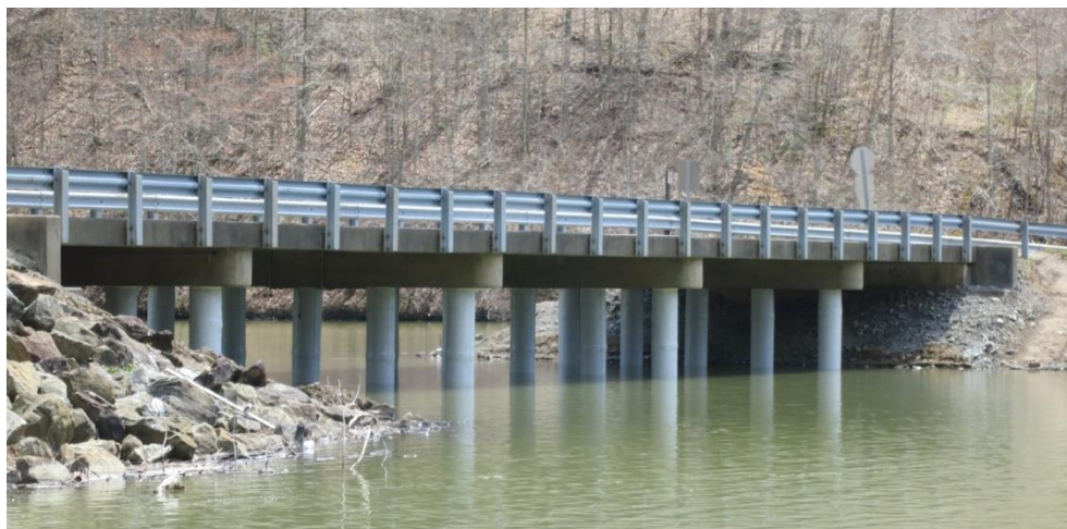
Figure 9.18 View of the bridge after rehabilitation, Photo by Dale Smith.
