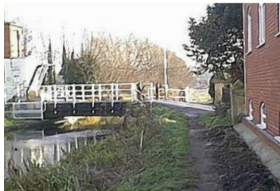
Figure 2.13 Bonds Mill bridge (UK, traffic bridge, 1994)
