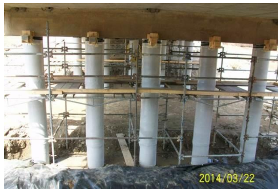
Figure 9.17 Columns with shells in placed and wrapped with GFRP wrap
