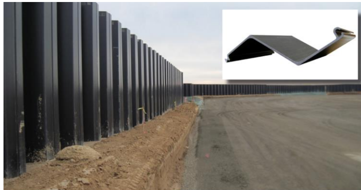
Figure 8.18 CMI'S UltraComposite™ UC 95 profile sheet piling for flood wall
