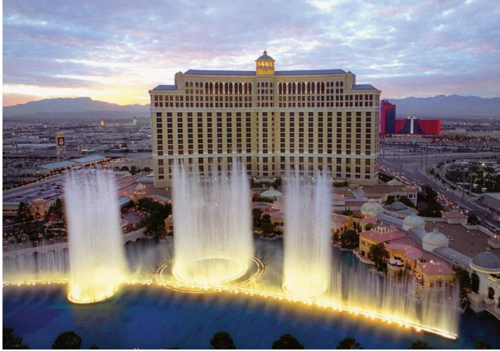
Figure 8.43 Bellagio Hotel and Casino fountain
