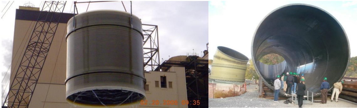
Figure 7.7 Large Diameter FRP Chimney Flue Liner (courtesy of International Chimney); Module liner section (left); connection elbow (right)
