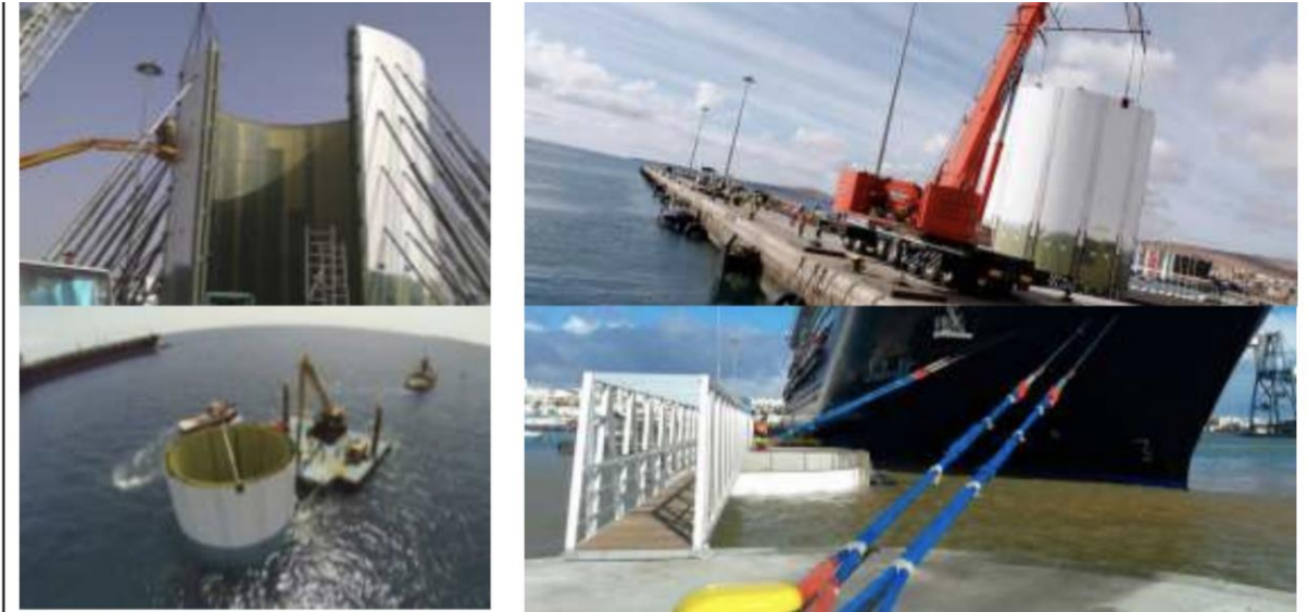
Figure 8.16 FRP Dolphin (Fuerteventura, Canary Islands-Spain,2014)
