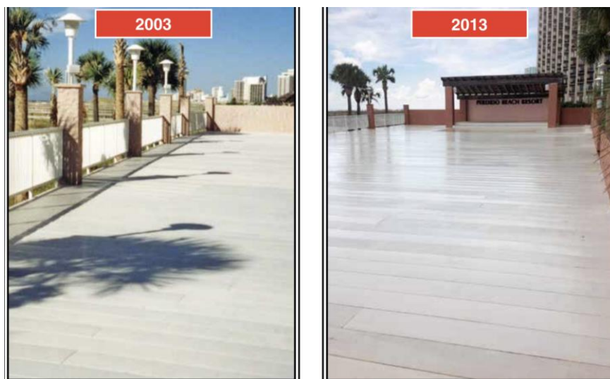
Figure 8.35 STRONGDEK™ installed at Perdido Beach Resort in Orange Beach, Alabama
