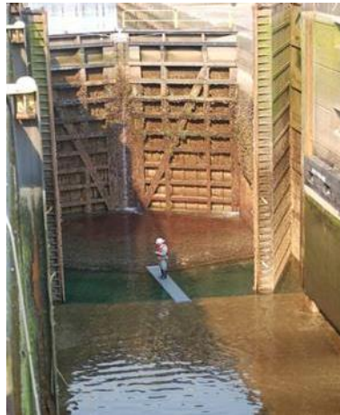
Figure 9.11 Miter gate
