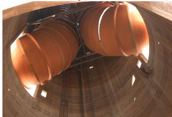
Figure 7.7 Large Diameter FRP Chimney Flue Liner (courtesy of International Chimney); Module liner section (left); connection elbow (right)
