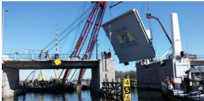
Figure 2.18 Elburgerbrug,, LM1 Traffic class FRP deck in existing lift bridge, (The Netherlands, 2015)
