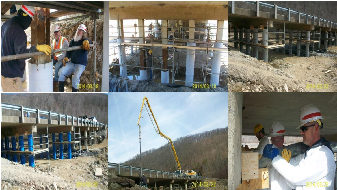
Figure 8.10 Rehabilitation Steps of Steel Piles with FRP Composites
