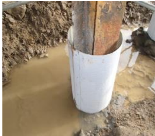
Figure 9.15 Close-up of shell placed around corroded steel pile
