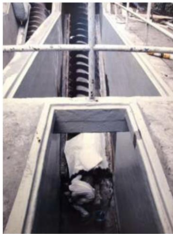
Figure 2.22 Coating of concrete structures with glass-fiber reinforced polyester
