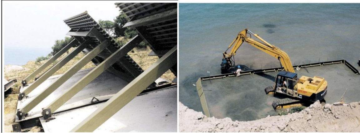
Figure 8.21 The Martin Beach Builder™, a new triangular framing system anchored to a precast concrete base
