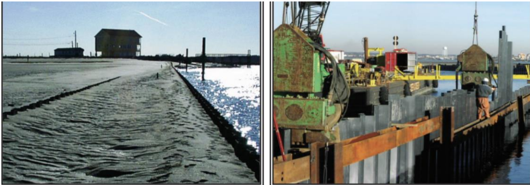
Figure 8.19 Walls made of UltraComposite™ UC 30 sheets
