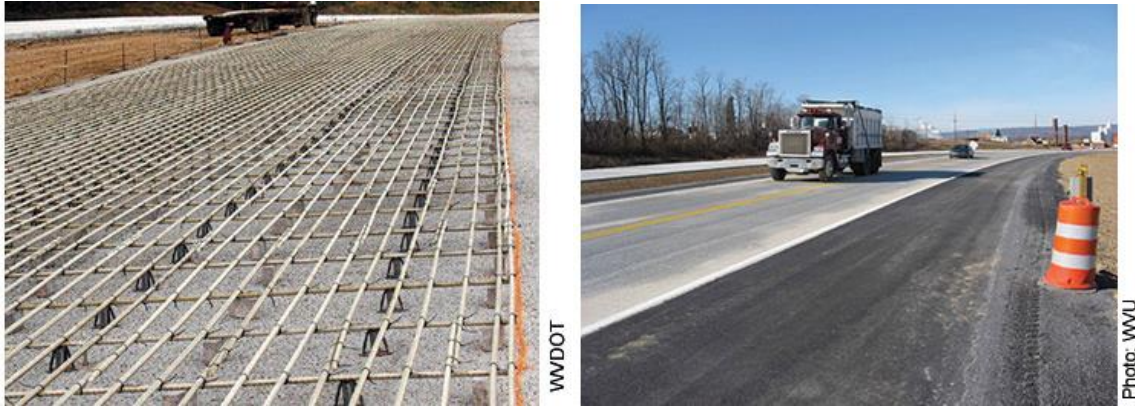
Figure 7.3 Pavement with FRP Rebar, WV Route 9, Martinsburg, WV (Chen et al, 2008)
