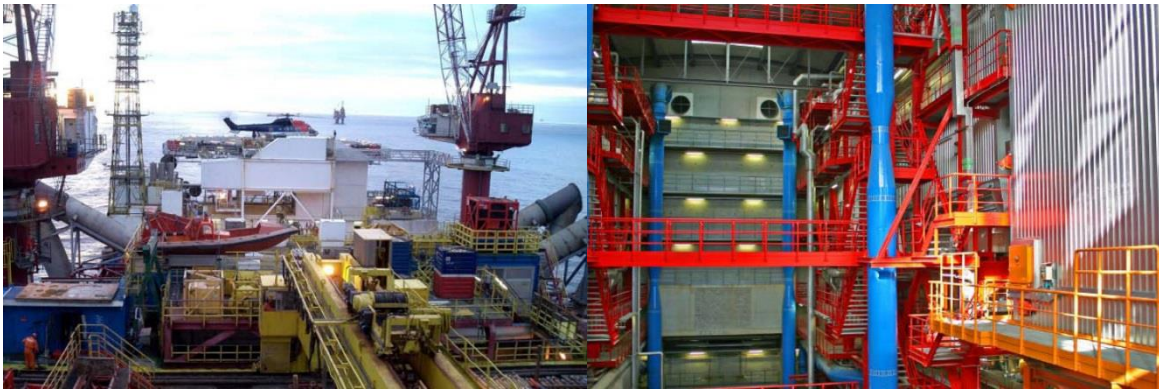
Figure 8.37 FRP Handrail, Ladder, Platform and Walkway for Sea Waterfront Facilities (courtesy of Bedford Reinforced Plastics Inc.)
