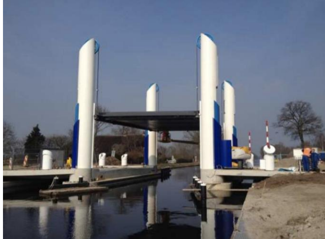
Figure 2.17 Pijlebridge, Meppel, LM 1 traffic bridge, (The Netherlands, 2015)
