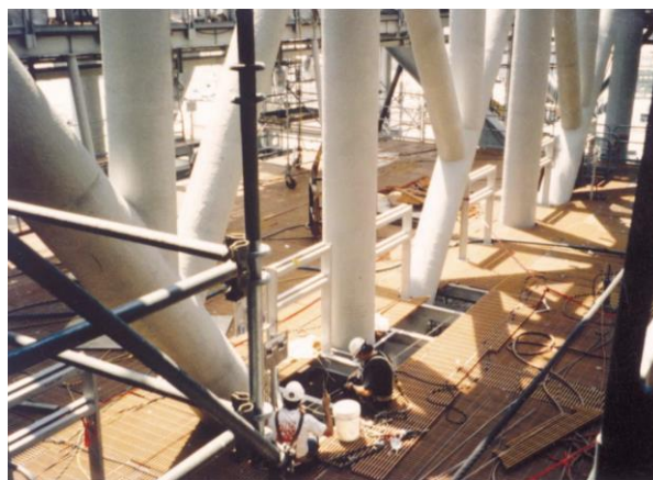
Figure 8.30 DURAGRID® phenolic grating used in Shell Mars tension leg platform in the Gulf of Mexico
