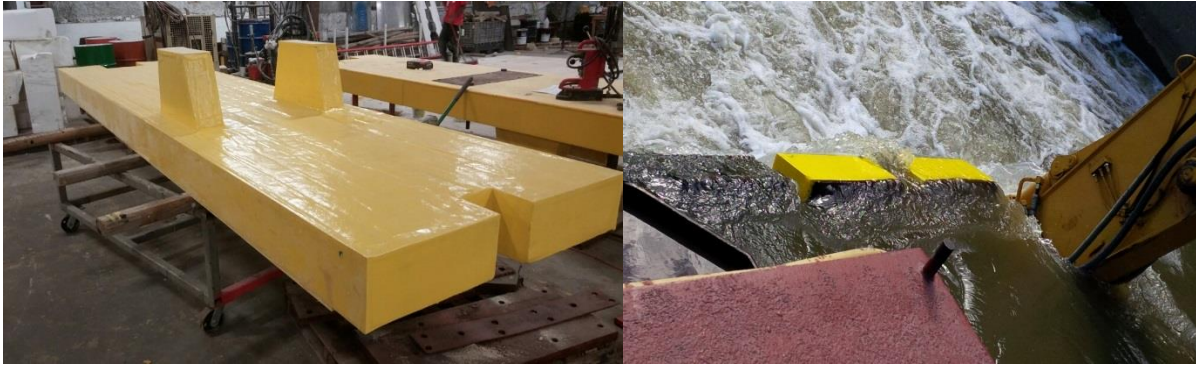
Figure 8.7 Composite Wicket Gates in Service
