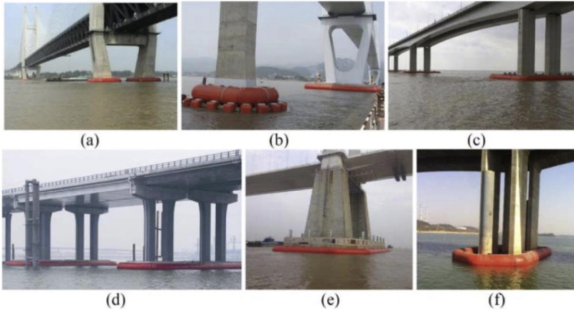
Figure 8.39 Applications of LCBS on bridge protection projects in China
