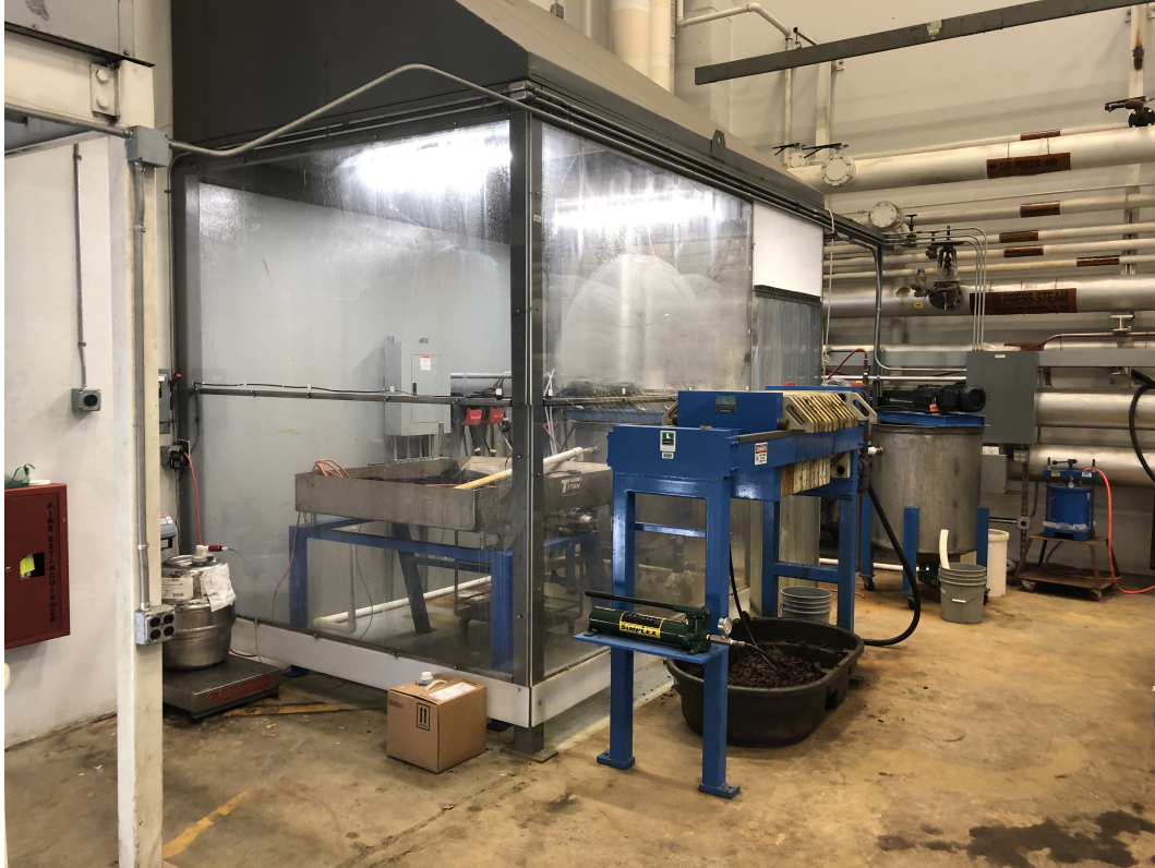
Figure 5.3 – Acid leaching module of bench-scale plant
