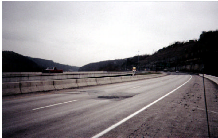
Figure 5.3: Photograph of Bridge #2667, I-79 North
