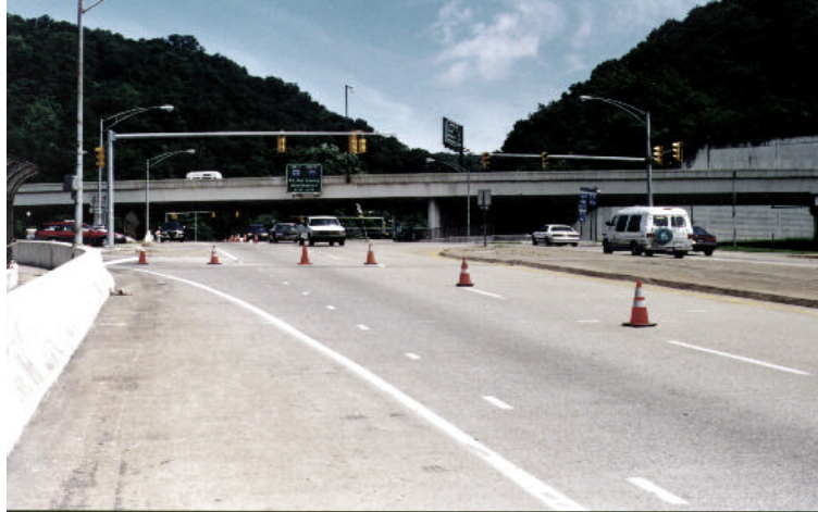
Figure 7.1: Photograph of Greenbrier Bridge
