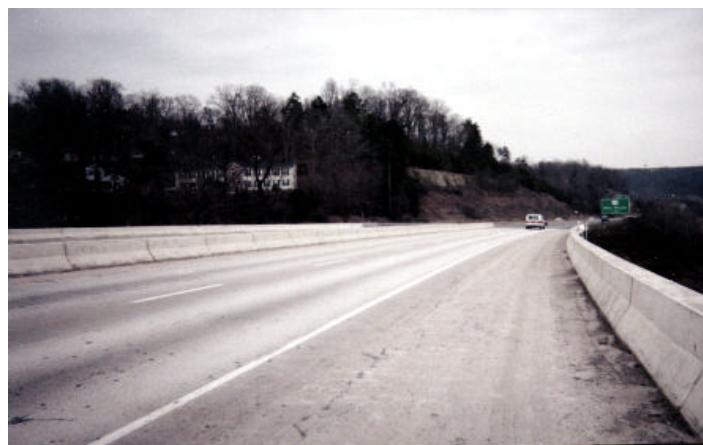
Figure 5.3: Photograph of Bridge #2667, I-79 South
