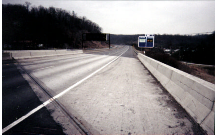
Figure 5.1: Photograph of Bridge #2666, I-79 North
