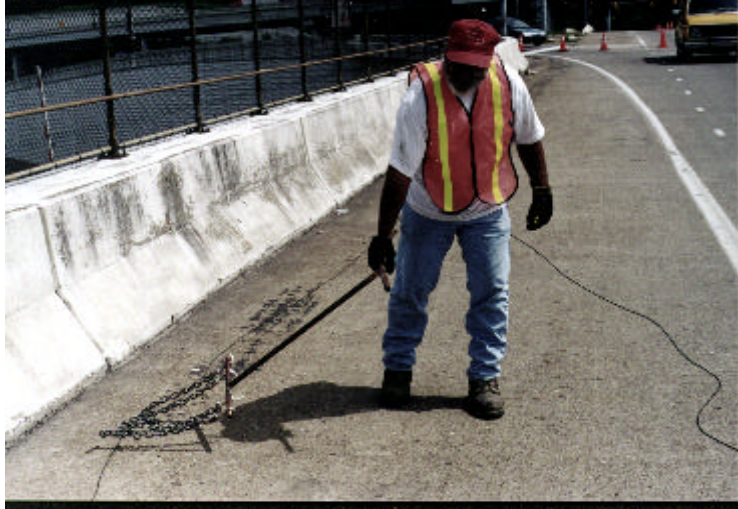
Figure 2.2: WVDOT Employee Conducting Chain Drag Test
