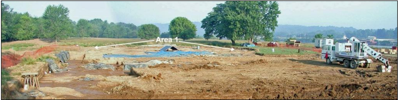
Figure 29: View of Area 1 (background) and Pier 5 excavated to near the top of CS II, facing slightly right of downriver (west-northwest). Photo taken 24 June 2003.
