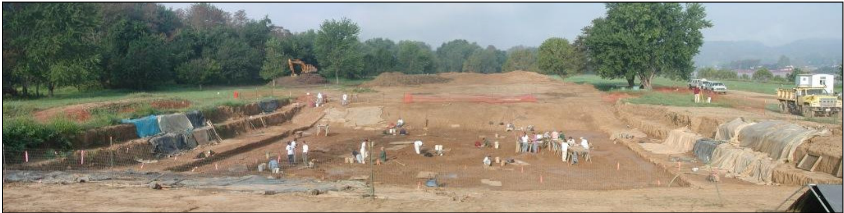
Figure 30: View of Pier 5 excavated to near the top of CS IV, facing downriver (west) on 7 September 2003.
