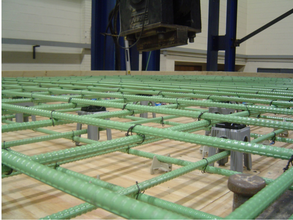
Figure 3.14: Typical top layer of rebar
