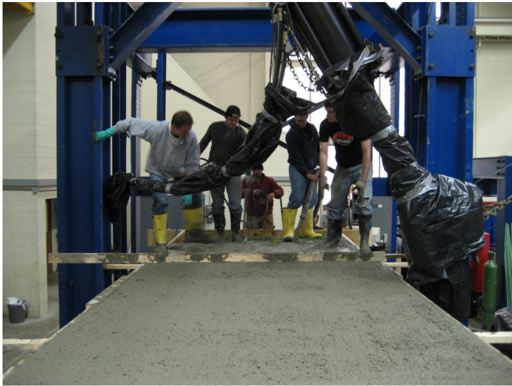
Figure 3.16: Concrete pouring process
