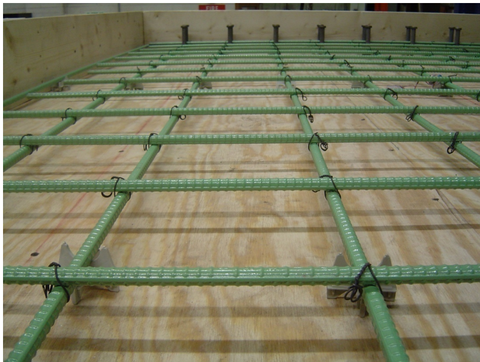
Figure 3.13: Typical bottom layer of rebar
