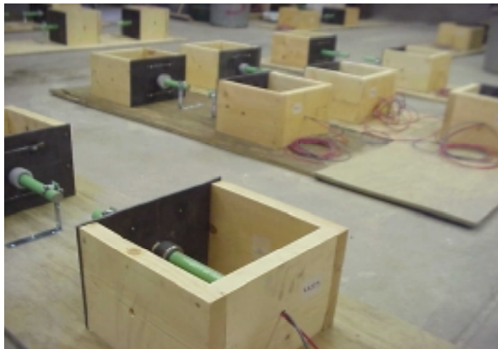
Figure 3.6 - A number of prepared molds ready to cast end sections
