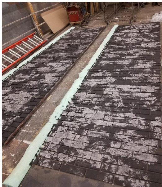
Figure 9.1 Based Black Homasote Bricks with Textured Applied on Top
