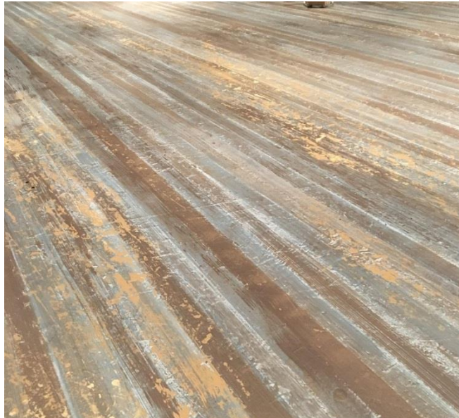
Figure 9.10 Final Paint Treatment
