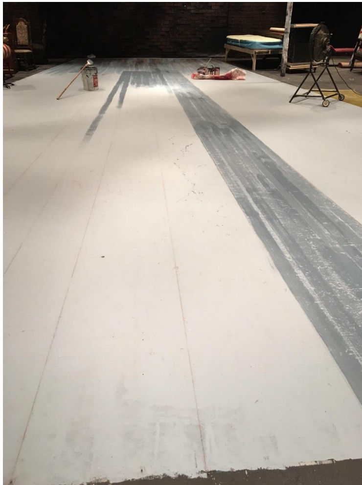
Figure 9.8 First Layer of Base Paint for Wood Planks
