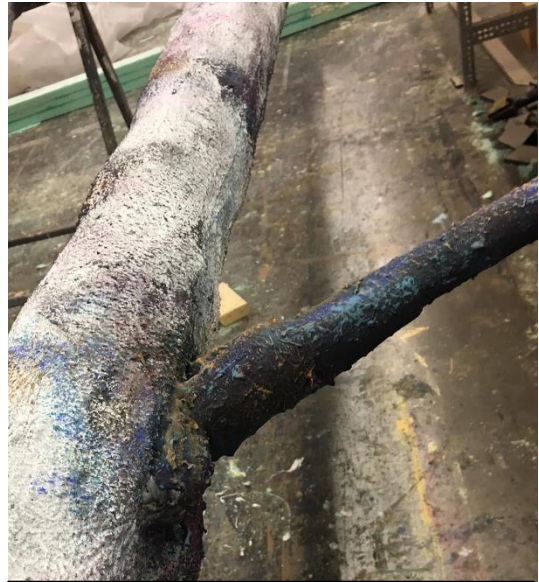
Figure 7.4 Final Paint Treatment
