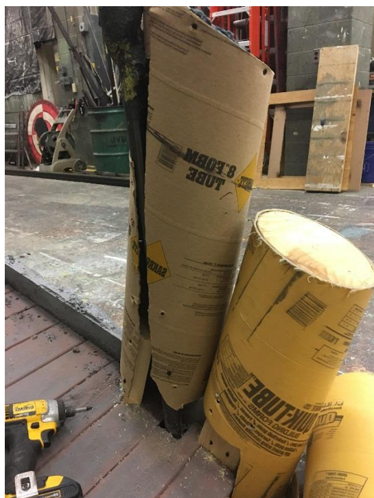
Figure 10.5 Beginning Process of Sonotube Tree Stumps
