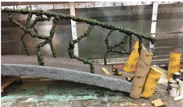
Figure 10.4 Texture and Paint Treatment on Steel Railings
