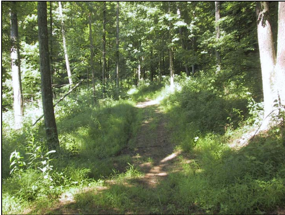
Figure A.2. Good application of outsloping on a skid trail.
