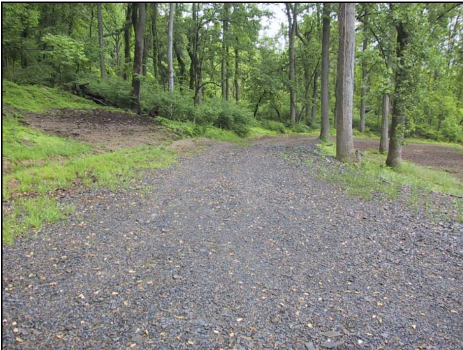
Figure A.4. Good application of gravel applied to a haul road.
