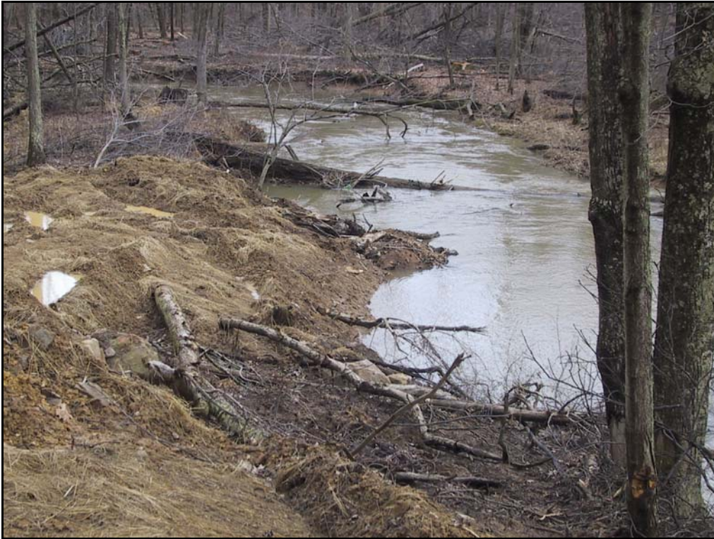
Figure A. 5. Poor application, effectiveness, and compliance of reclamation in a SMZ.
