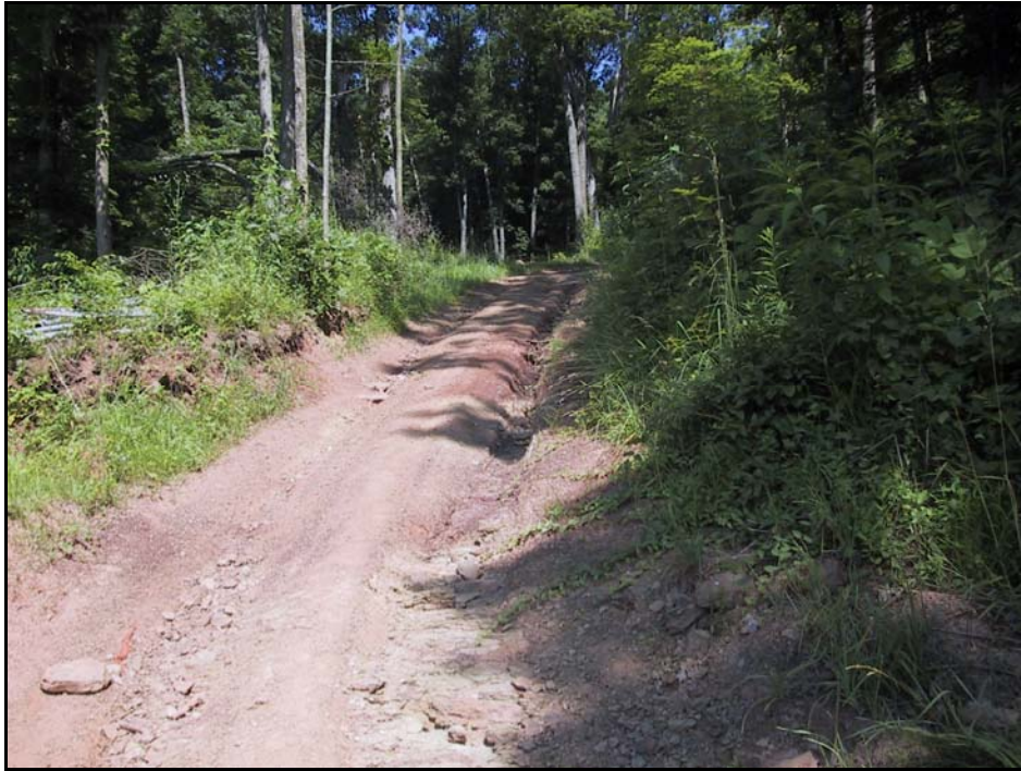
Figure A.1. Poor application of waterbars on a skid trail.
