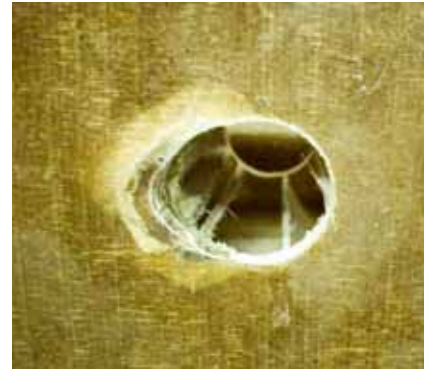
Figure 2.16 Delamination of Bottom Facesheet
