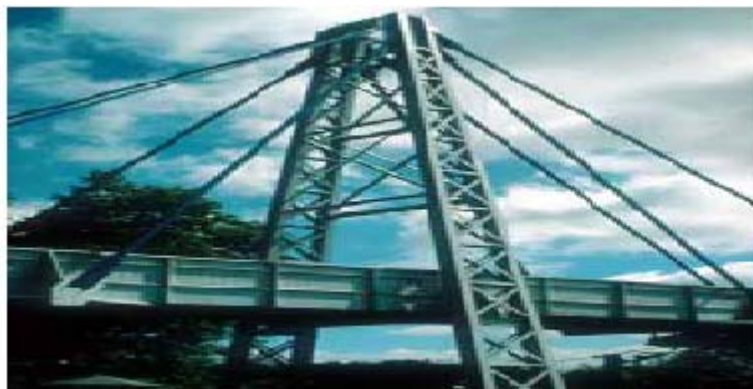
Fig. 1.1 All-Composite Foot Bridge in Kolding, Denmark. Erected in 1997 [Herbert (2004)]
