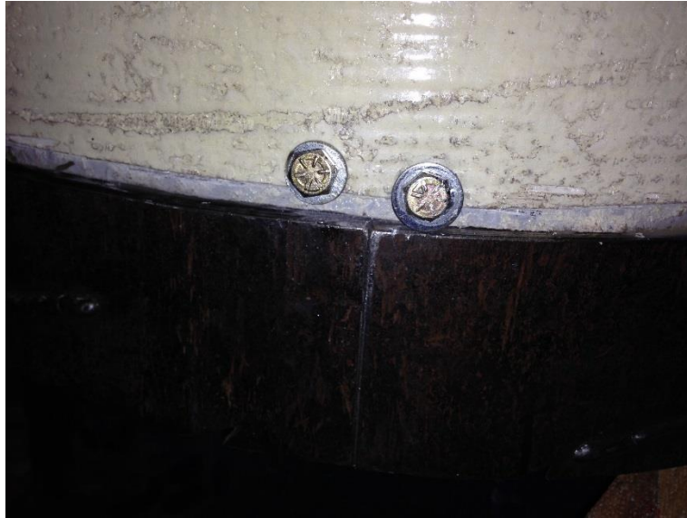
Figure 4-7: Auger adjoined to the FRP shell with bolts and Epoxy.
