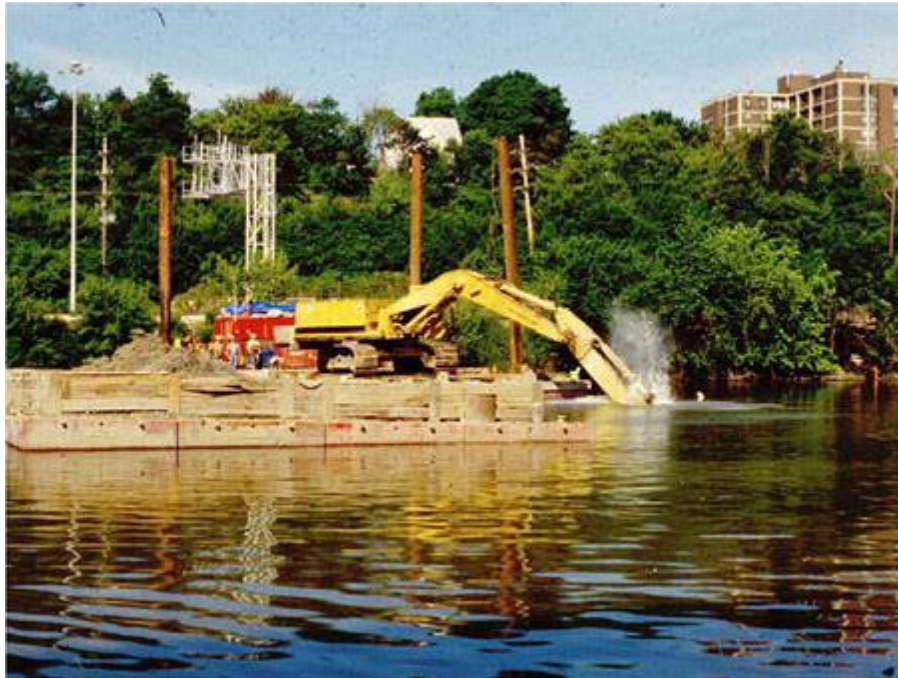
Figure 2-7: Excavator (ABC Diving® , 2016).
