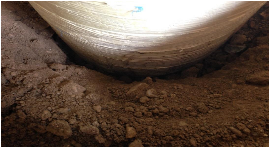
Figure 4-16: The FRP shell going down as soil is pushed aside.
