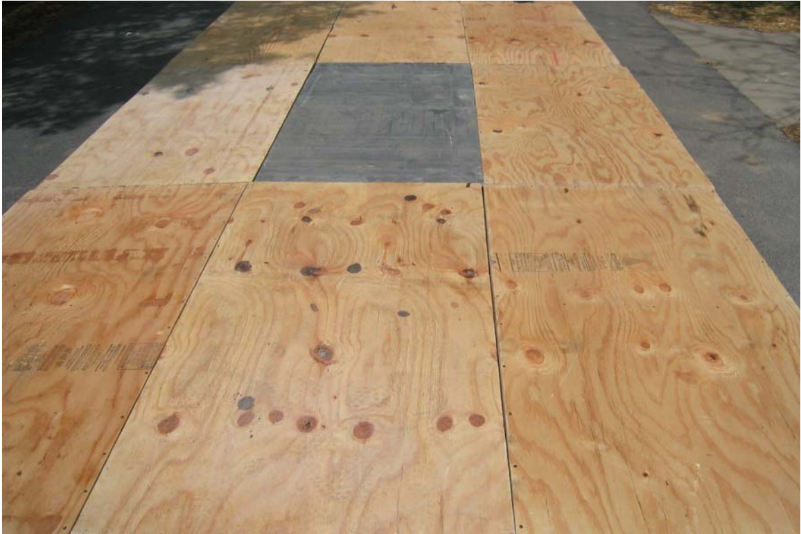
Figure 7.5: FRP Deck module with the wooden platform setup.
