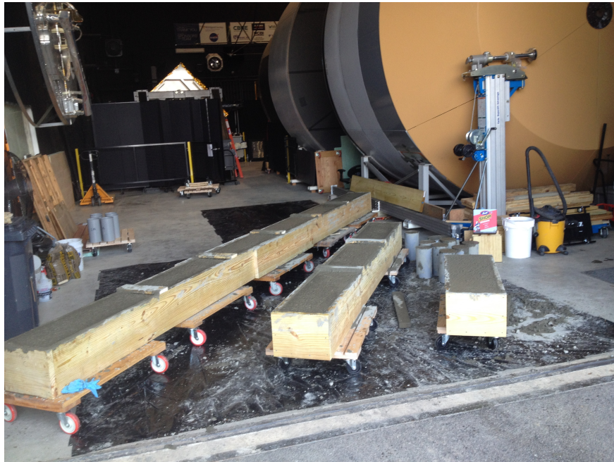
Figure 3.2: Concrete Beams Immediately After Pour. From Left to Right: 6 m, 3 m, and 1 m beams
