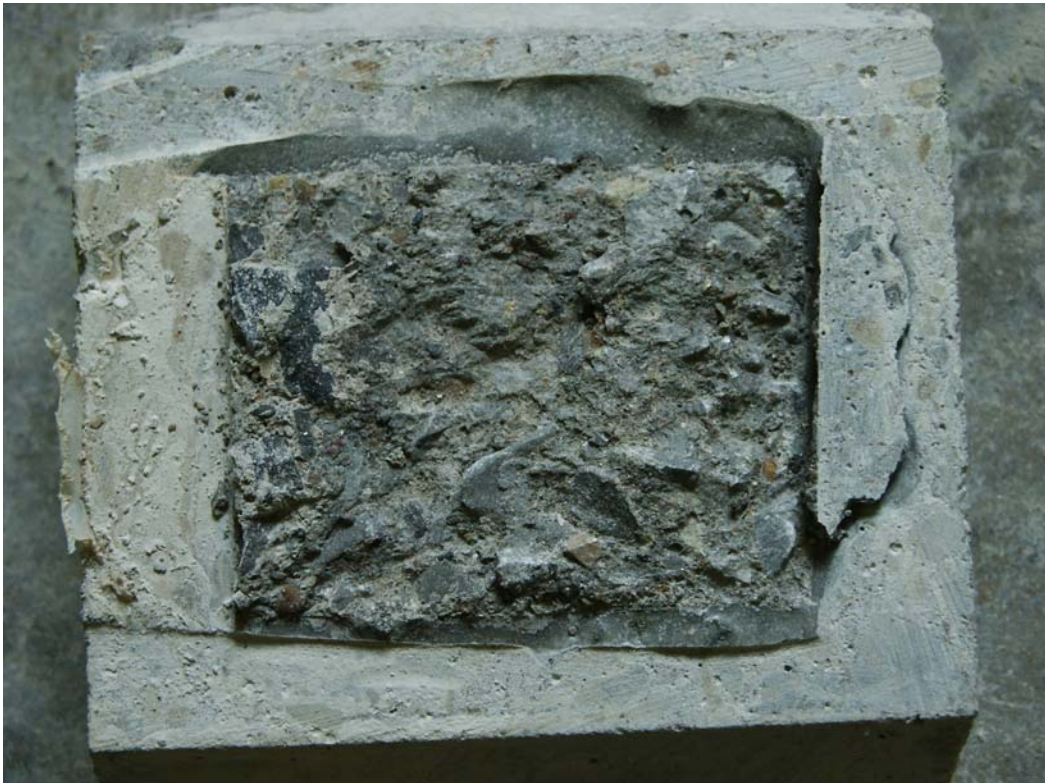
(d) Failure of Surface Preparation CSP #8 (Enlarged View)
