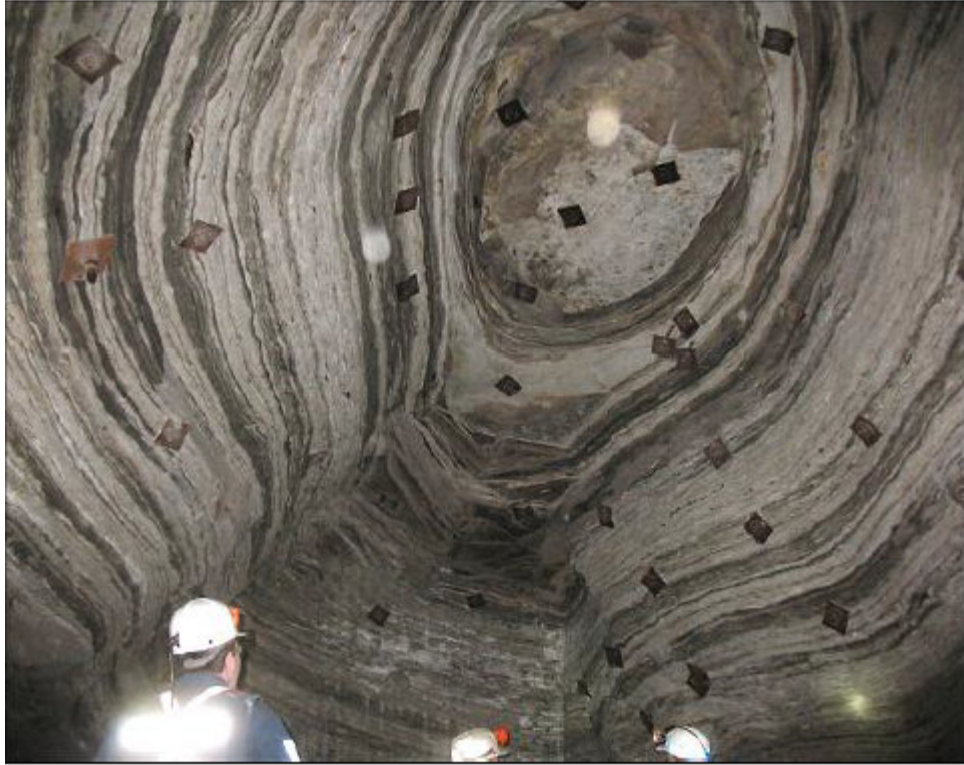
Figure 2.6 Dome-shaped cavity caused by progressive failure of interbedded shale and sandstone roof at a mine located in Illinois (Esterhuizen and Bajpayee, 2012).
