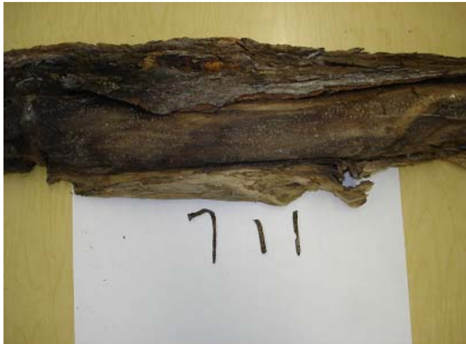
Figure 5-36 Rotten piece and metal nails extracted out from Log 3
