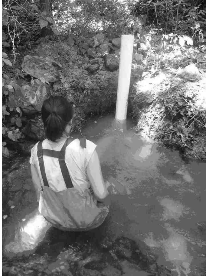
Figure 6. Installing stilling well at Rock Gap Run, July 2006 (photo Matt Finkenbinder).
