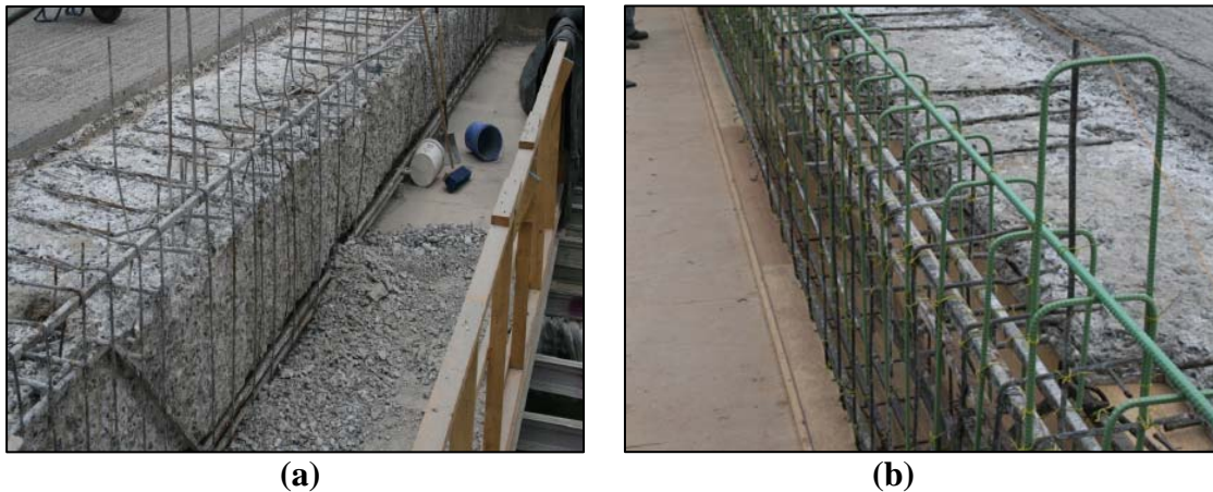
Figure 6.1 Concrete Demolition – (a) Beam 1 (b) Beam 6
