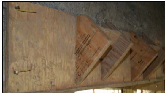
Figure 6.5 Patch Formwork Detail
