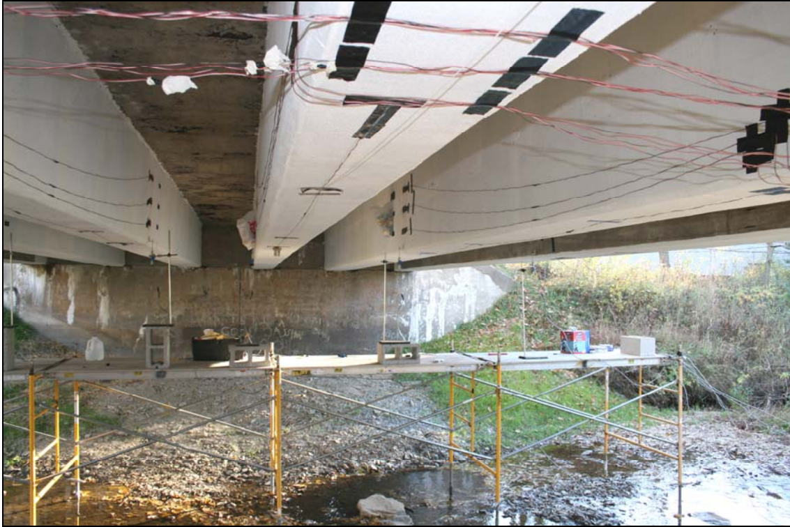
Figure 3.8 Overall Test Setup
