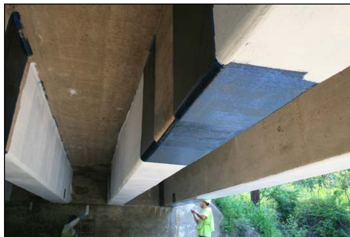
Figure 6.9 FRP Reinforcement Layout for Beams 2 & 3
