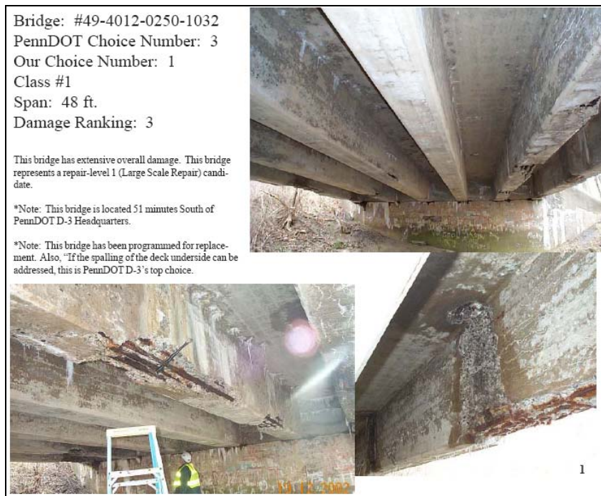
Figure 1.3 Bridge Condition Photographs
