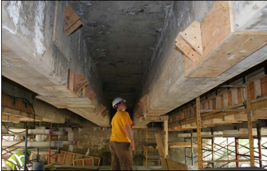
Figure 6.4 Patch Repairing Formwork along Beams 3 & 4
