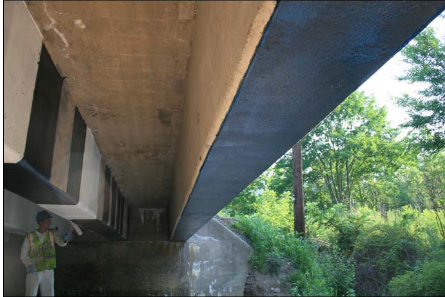
Figure 1.4 Beam 1 and 2 FRP Reinforcement
