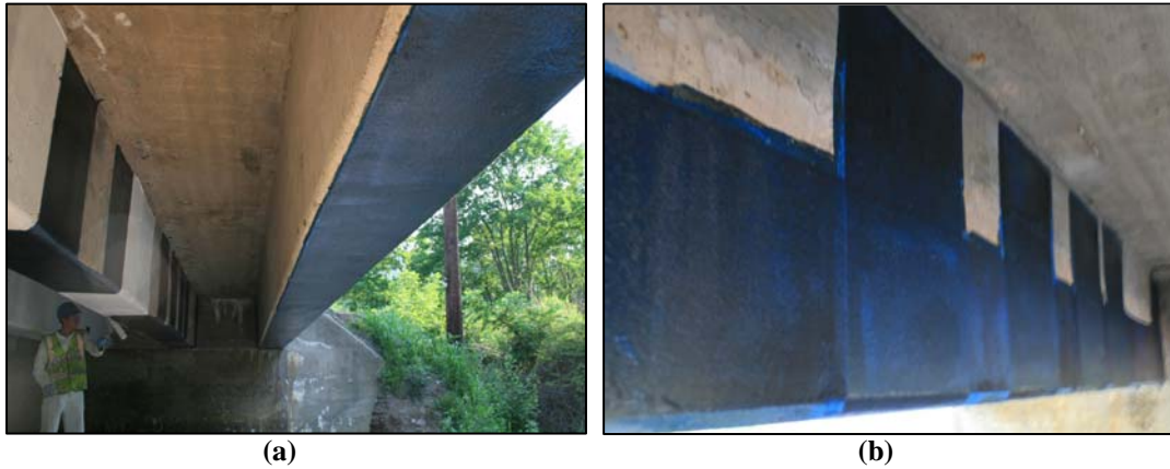
Figure 6.8 FRP Reinforcement Layout (a) Beam 1 & (b) Beam 5
