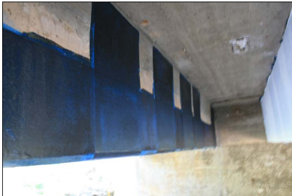
Figure 1.5 Beam 5 FRP Reinforcement
