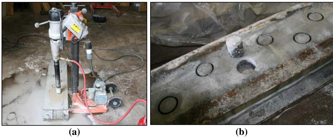
Figure 6.14 Concrete Pull-Off Test (a) Drill Setup (b) Tested Core
