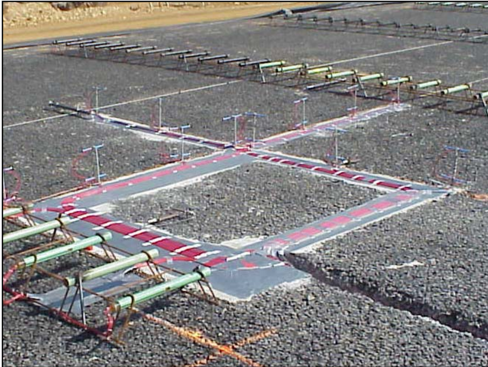
Figure 4.2 Typical Slab Instrumentation Prior to Concrete Placement.
