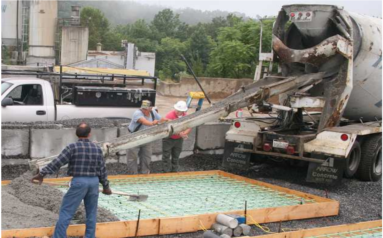
Figure 3-1 Mixing truck, and placing
