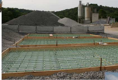
Steel Placement & Instrumentation
