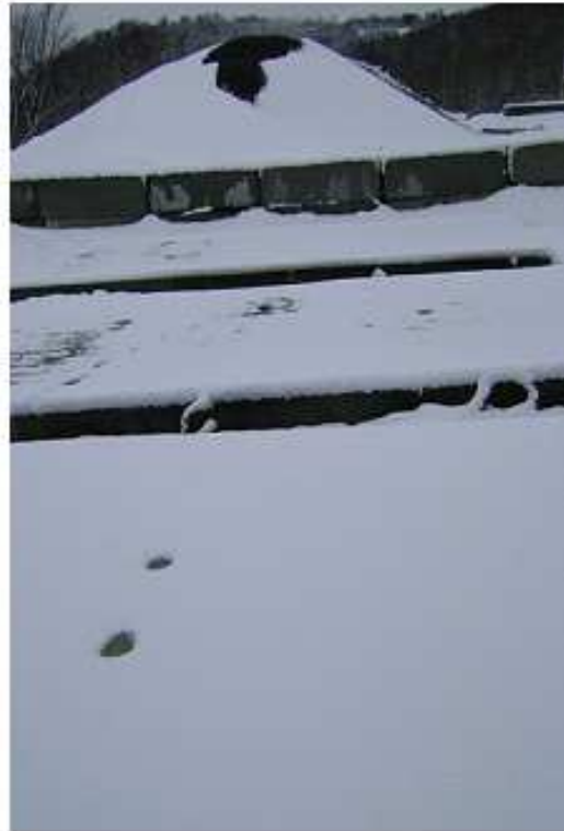
90 Days After Pouring
