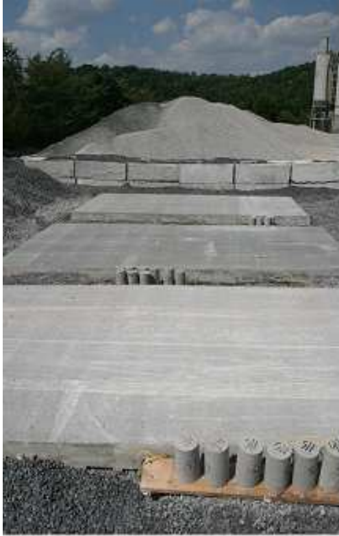
10 Days After Pouring
