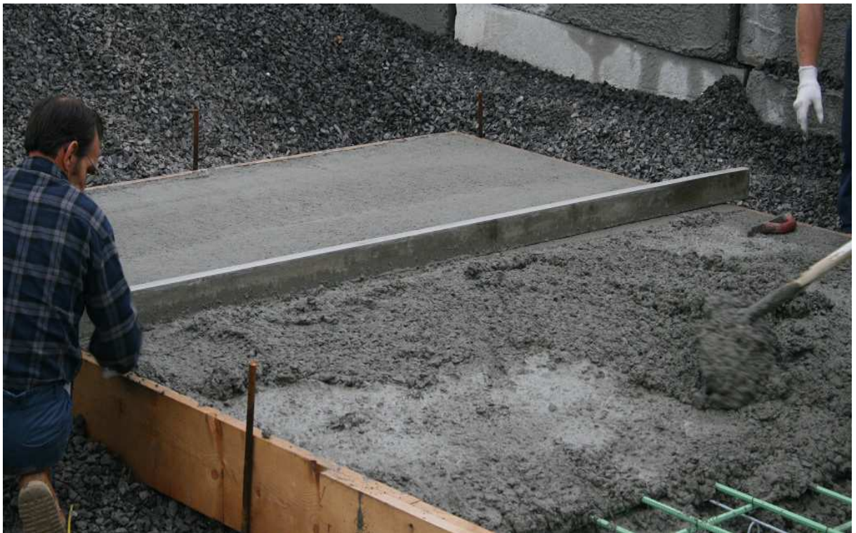
Figure 3-2 Leveling placed concrete
