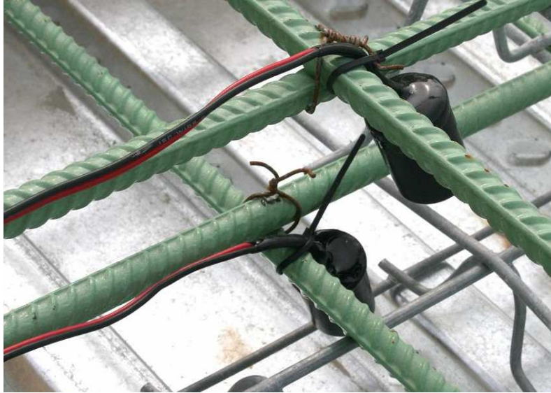
Figure 5-3 Maturity Loggers Attached to the Top and Bottom Steel Reinforcement
