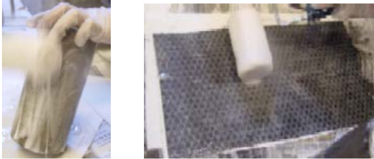
Figure 4-10 Impregnating with Epoxy
