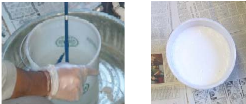
Figure 4-9 Mixing of Epoxy and Hardener
