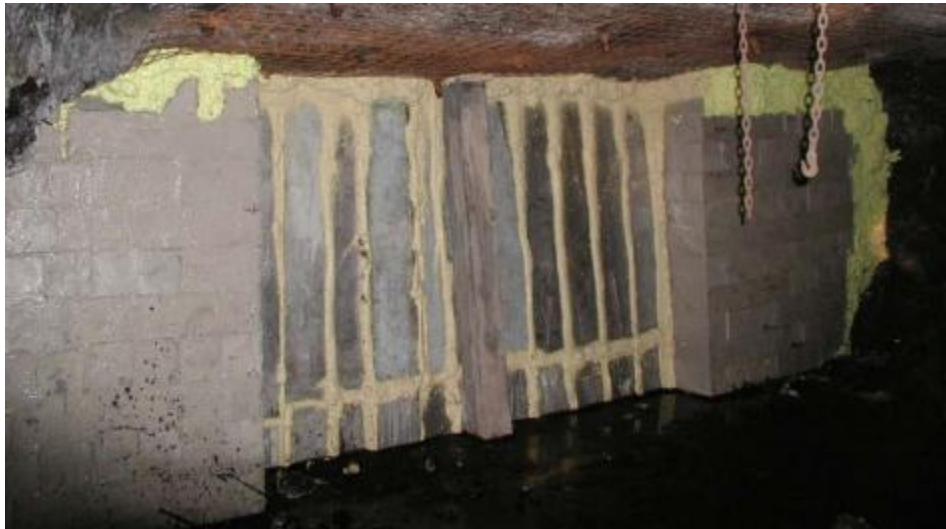
Figure 3.3 Gob seal constructed with steel Kennedy panels and Omega blocks (Stephens, 2011)
