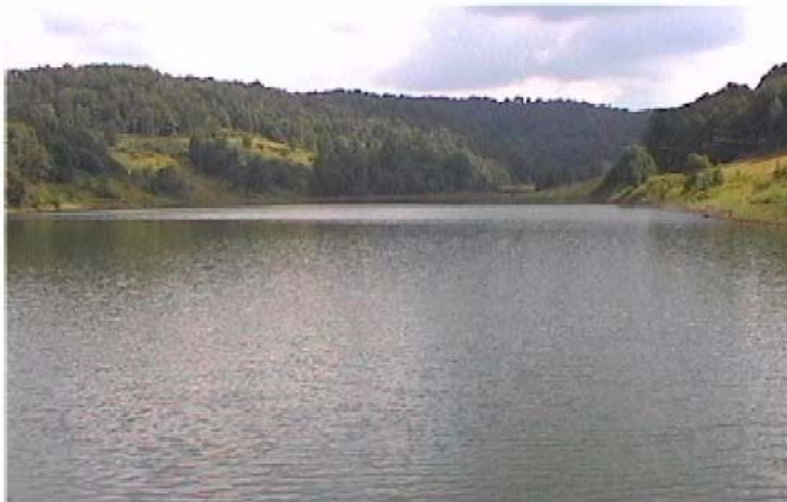
Figure 2.4 Photograph of Solids Settling Pond.
