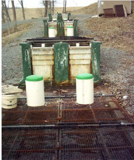
Figure 3.8 Photograph of Demand Feeders Installed on Each Raceway Segment.
