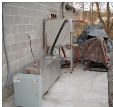
Figure 17: New concrete pad and system cooling equipment.
