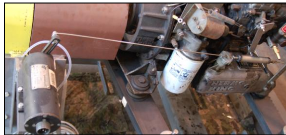
Figure 22: Servo motor and fuel rack control linkages.
