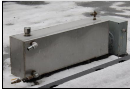
Figure 11: Immersion heater housing tank.
