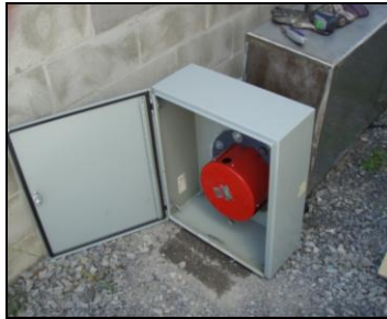
Figure 13: Chromalox immersion heater within tank.
