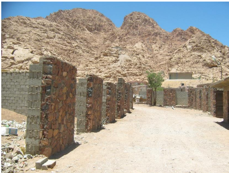
Ongoing construction of retail space downtown Katriin
