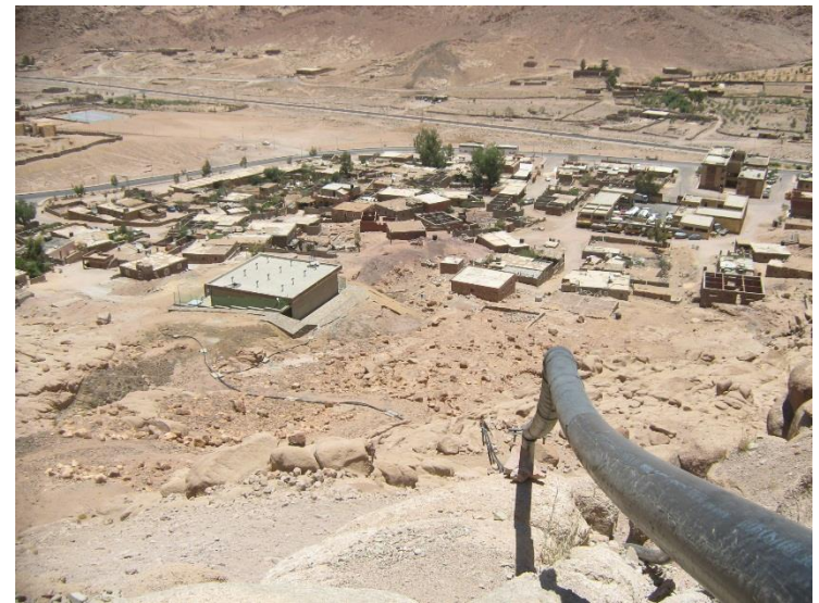
View of Shameya and the new water tower from the old Israeli tank
