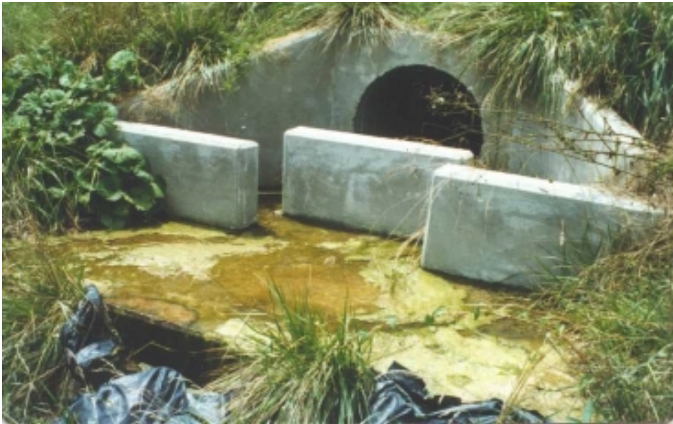
Figure 1.4.1 First Example of a Typical Standard Baffle Installation
