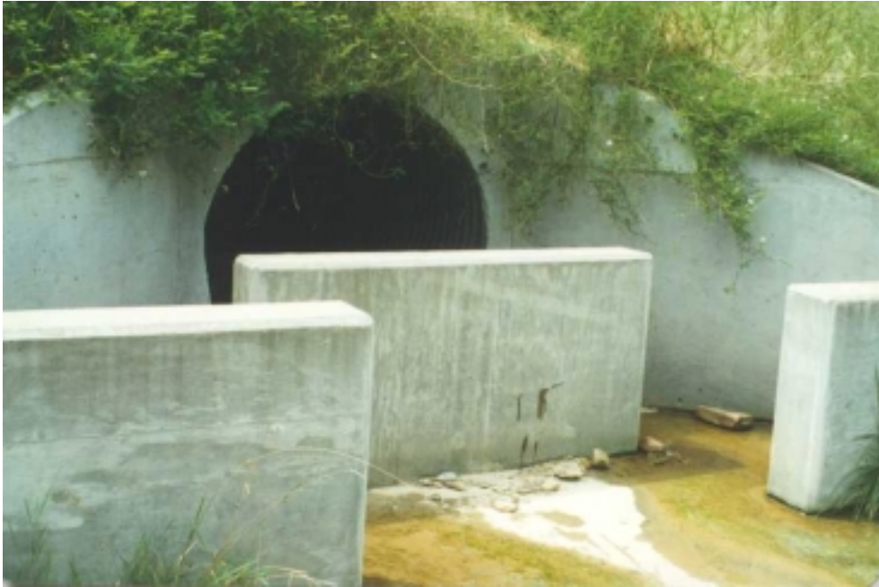
Figure 1.4.2 Second Example of a Typical Standard Baffle Installation
