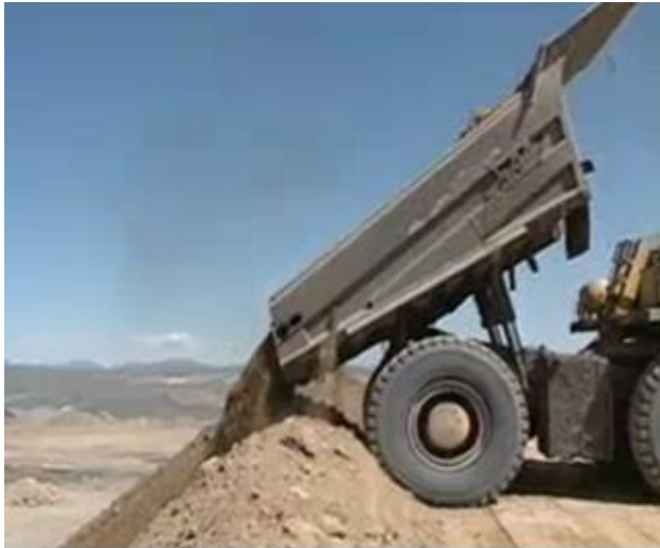
Figure 4.27 Safety berms along haul road and dump area (MSHA, 2014)
