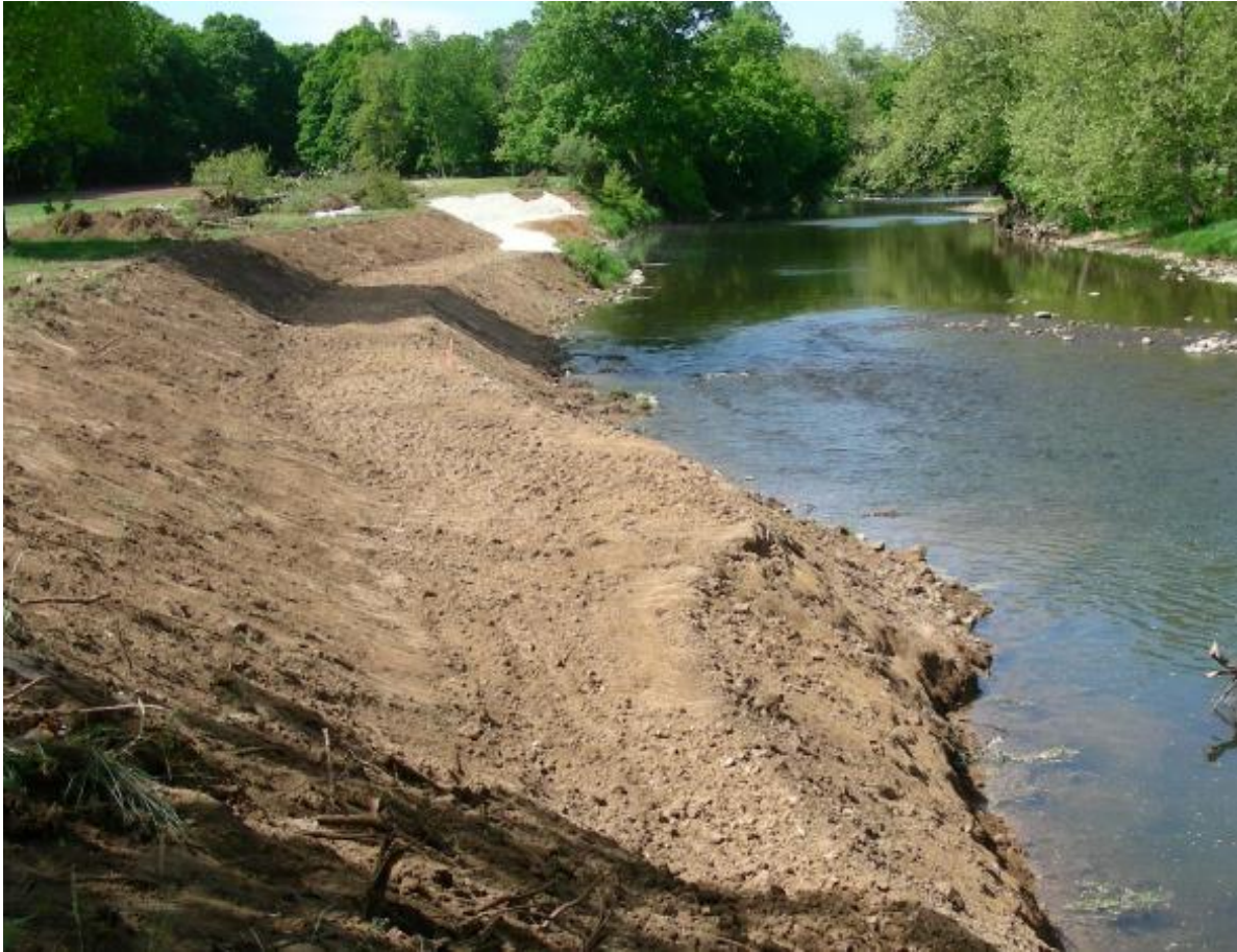
Figure 3. The eroded banks along the restoration reach were terraced to provide a gentler slope and small floodplain to decrease erosion and increase aggregation of sediment, taken May 2010.
