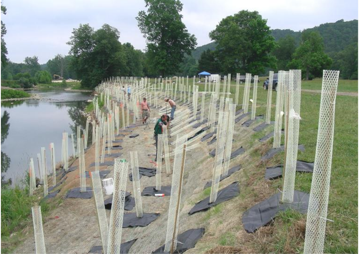
Figure 6. Trees and shrubs were planted on both sides of the restoration reach to re-establish the riparian zone and aid in bank stabilization. Tree tubes were placed around every sapling to prevent herbivory, taken June 2010.
