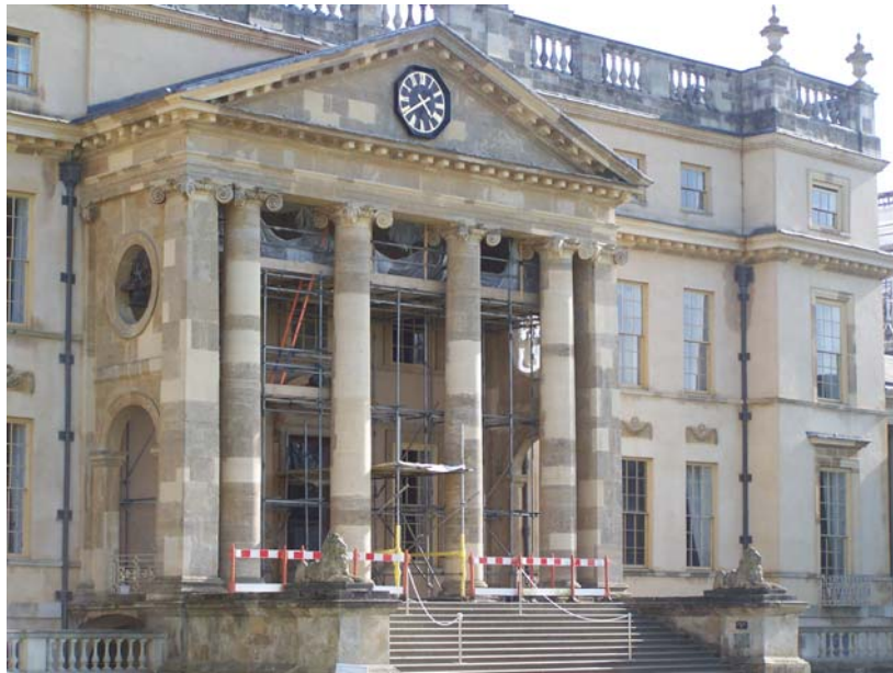
Figure 3. Close-up of North Front entrance.
