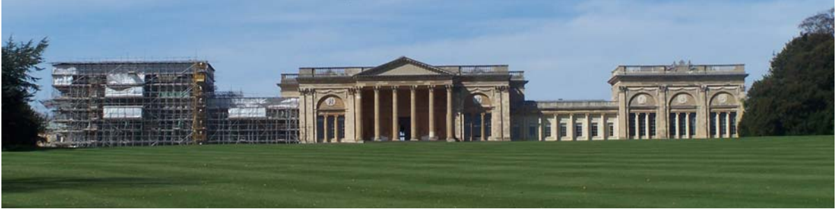
Figure 2. South Front of Stowe House.
