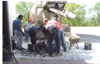
Figure 3.2b Pouring Uninstrumented Specimens
