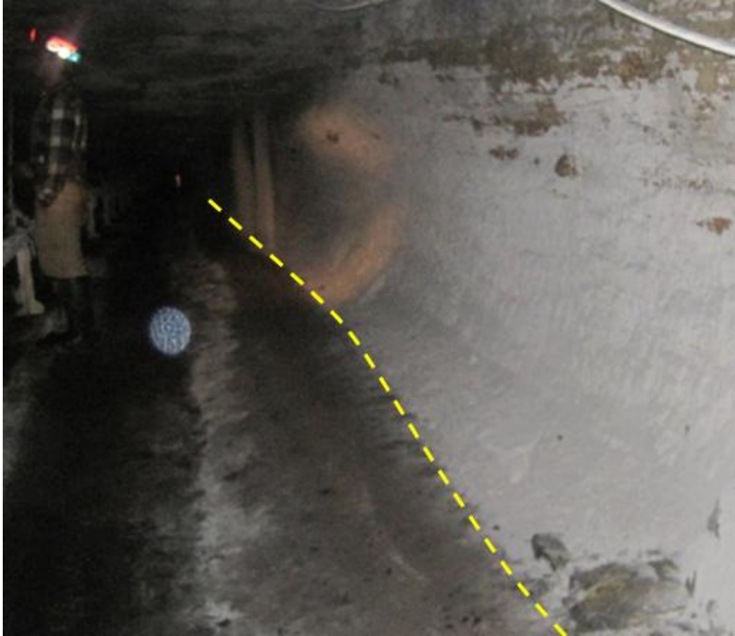
Figure 5.17 Subsidence up dip in the belt entry
