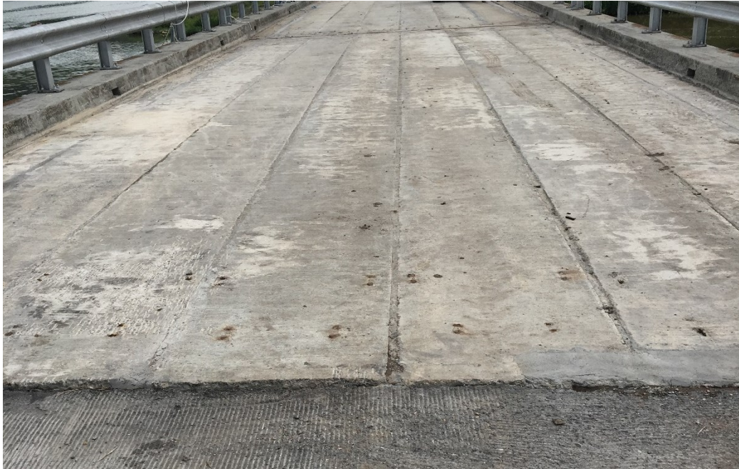
Figure 5-6: Wearing surface of the Whiteday Bridge under repair work
