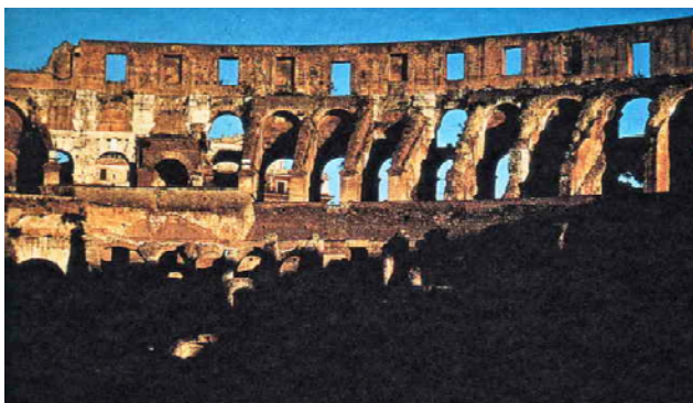
Plate 47. Graves, Flavian Amphitheatre, Colosseum, No. 1, Imperial Forums, Rome, Italy, 1961, Kodachrome (Photo by Michael Graves)
