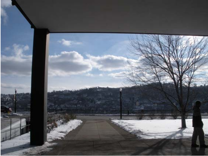
Plate 30. Mies, Mellon Hall steel column or pilotis (Photo by author)
