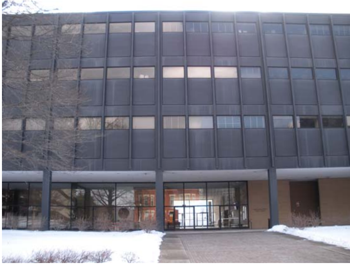
Plate 17. Mies, Richard King Mellon Hall of Science, Pittsburgh, Pennsylvania, 1962-68 (Photo by author)
