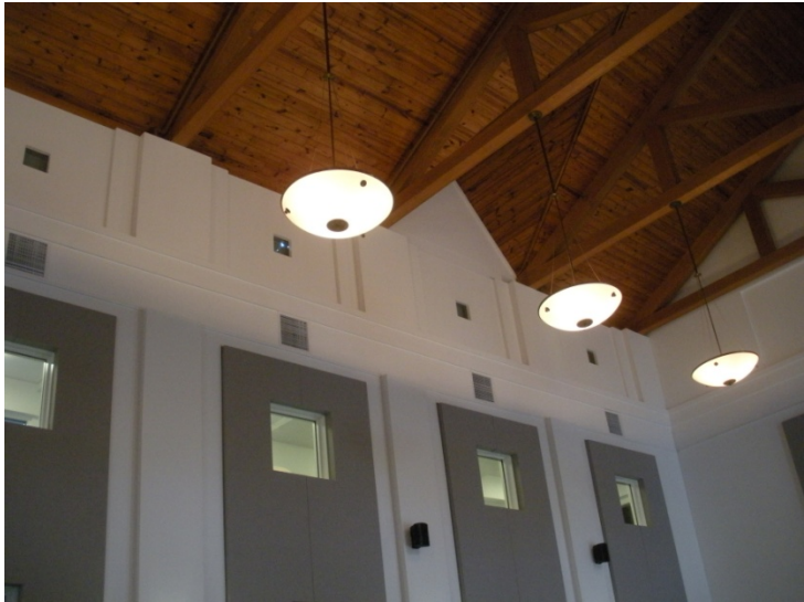
Plate 75. Erickson Alumni Center Great Hall ceiling beams and pedimental shapes, acoustic panels added later (Photo by author)
