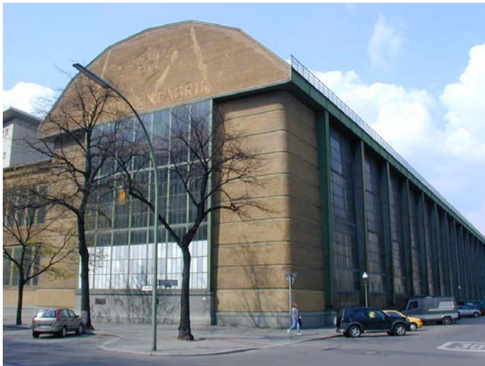
Plate 9. Peter Behrens, A.E.G. Turbine Factory, Berlin, Germany, 1908-09
