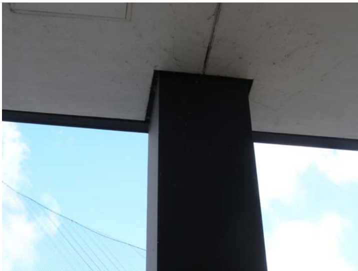
Plate 29. Mies, Mellon Hall steel column or pilotis (Photo by author)
