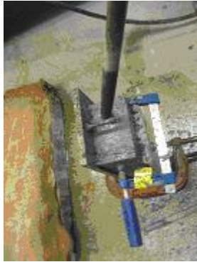
Figure 4.14 (d): Use of vibrating rod
