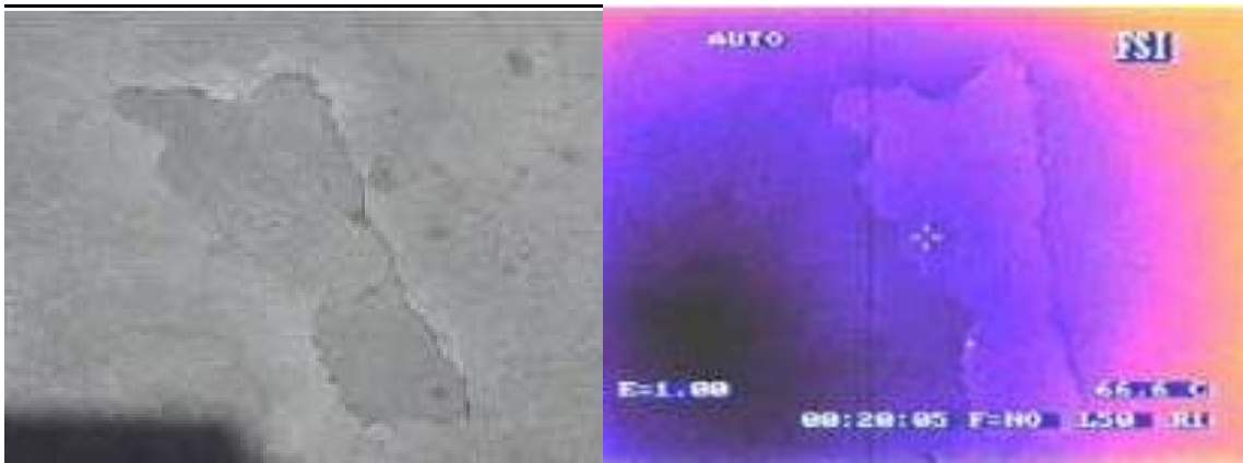
Figure 3.1.7 (a) Surface irregularity (Alqannah 2000). (b) Infrared image of the surface irregularity (Alqannah 2000).
