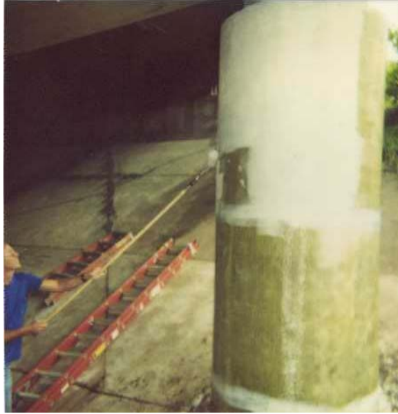
Figure 5.2.3. Resin is being applied on the column.
