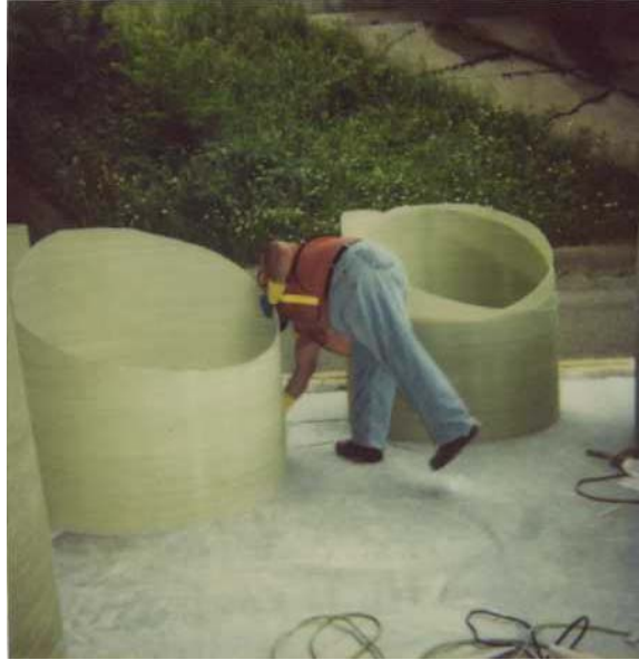
Figure 5.2.4. The pre-cured shells are ready for application.
