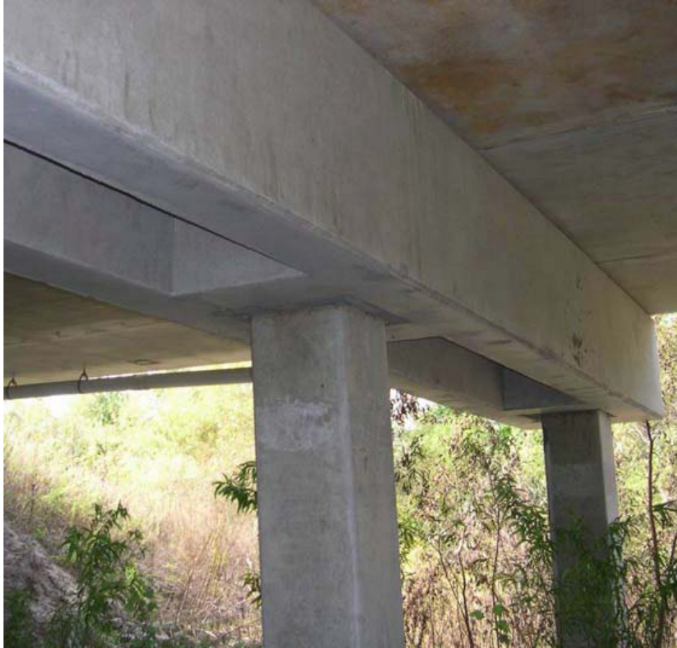
Figure 4-2 Precast Reinforced Concrete Bent Cap [14]
