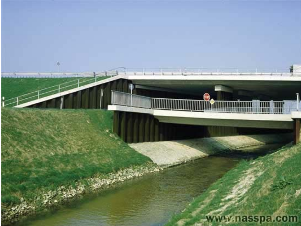
Figure 4-16 Steel Sheet Pile Wall Abutment [36]
