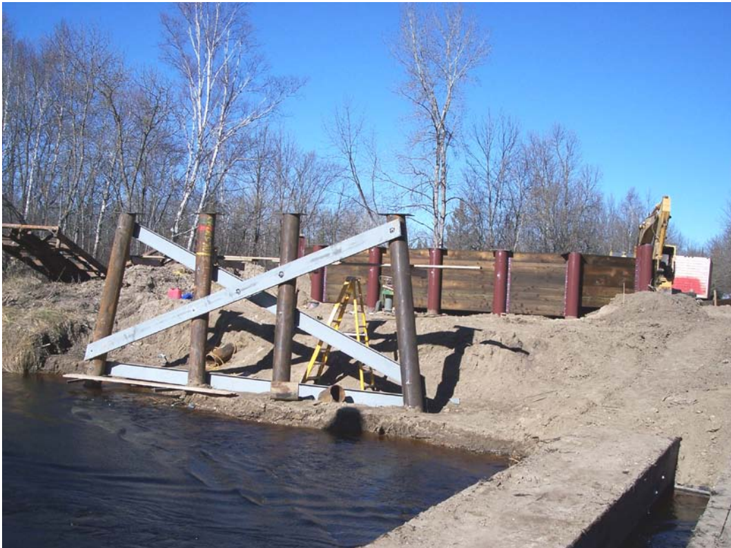
Figure 4-12 Driven Steel Piles for Piers/Abutments [12]
