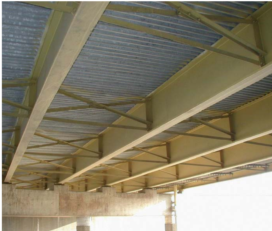
Figure 4-23 Steel Plate Girders as Bridge Superstructure [11]
