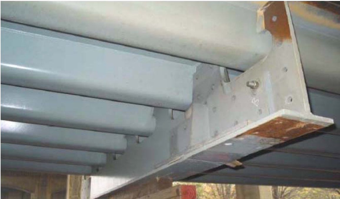
Figure 4-35 Underside of Steel Orthotropic Deck [25]
