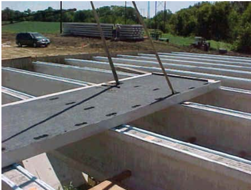
Figure 4-32 FRP Deck Panel Installation [22]
