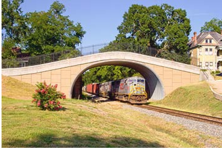
Figure 4-20 Corrugated Structural Plate as a Bridge Superstructure [9]
