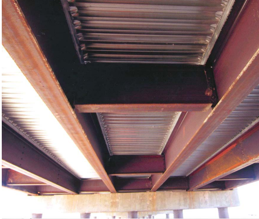
Figure 4-58 Bridge with Steel Diaphragms [31]
