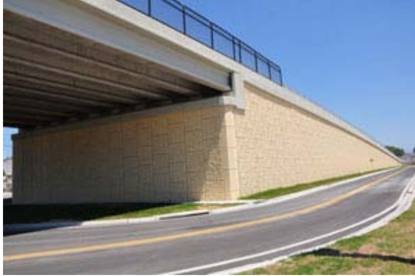
Figure 4-5 Mechanically Stabilized Earth Wing Wall [28]
