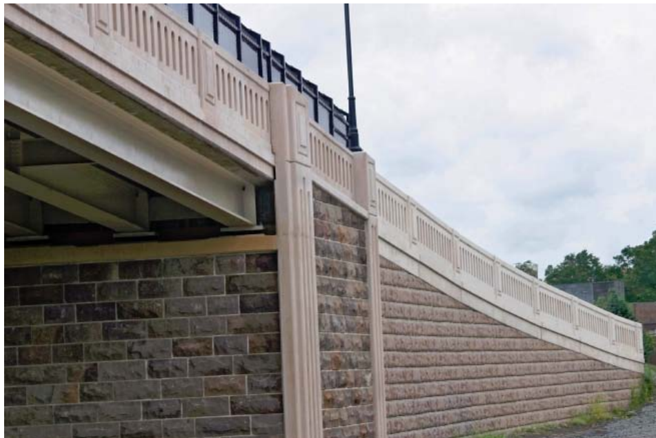
Figure 4-8 T-WALL® Wall System Installation [33]
