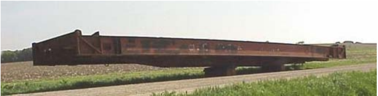
Figure 4-48 Decommissioned Railroad Flat Car Trimmed for Use as Bridge Superstructure [57]
