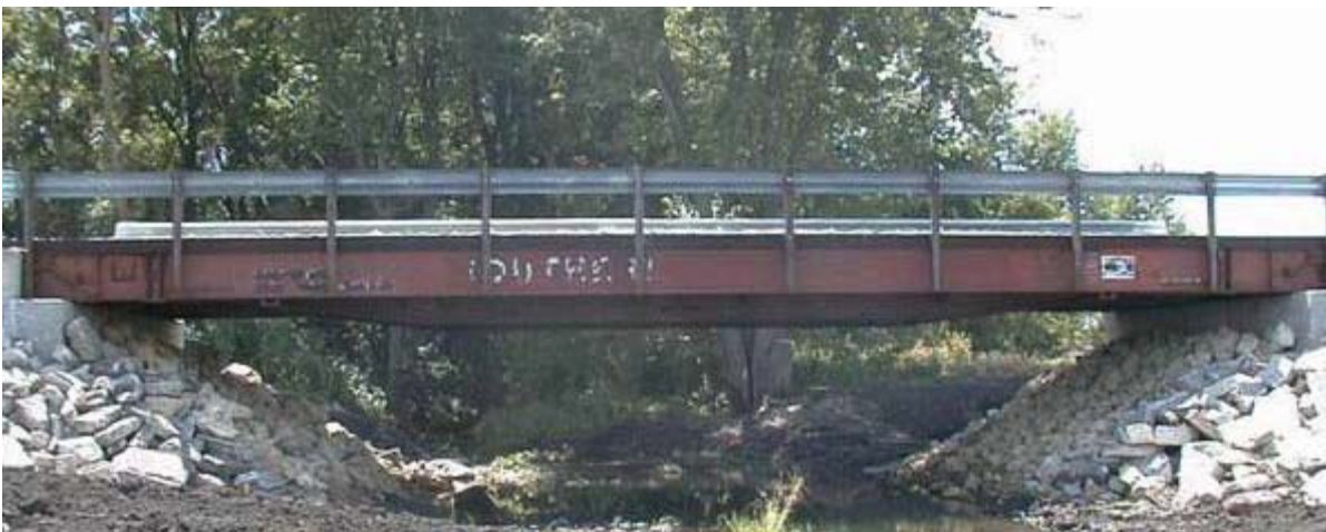
Figure 4-49 Side View of Railroad Flatcar Bridge [57]
