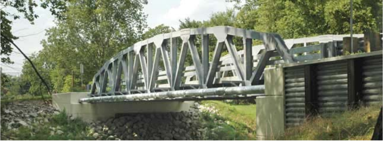
Figure 4-24 Cambridge Steel Truss Bridge [47]
