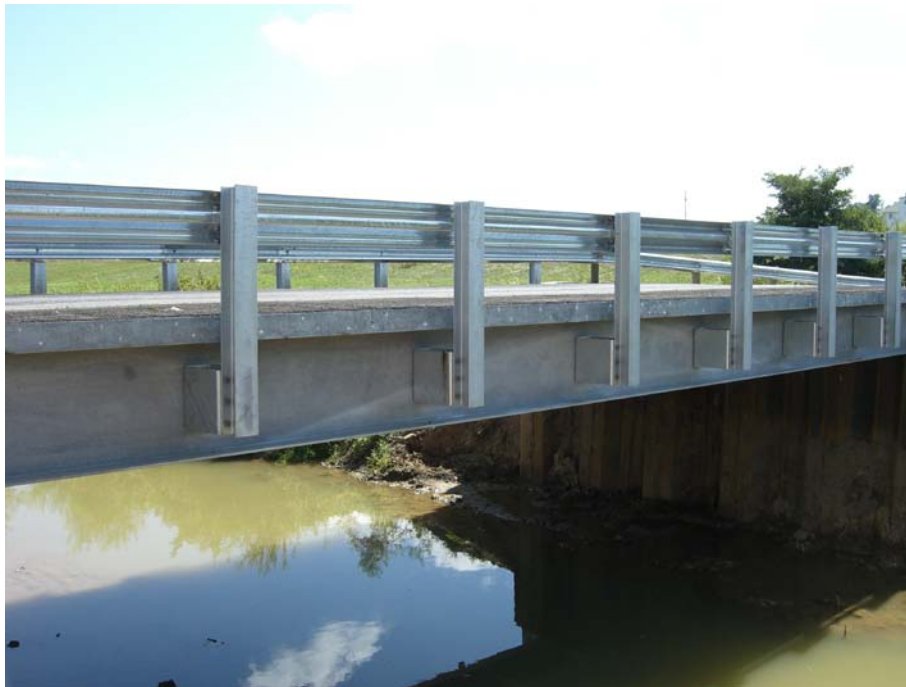
Figure 4-53 Steel Beam Rail Barrier (U.S. Bridge Tour)
