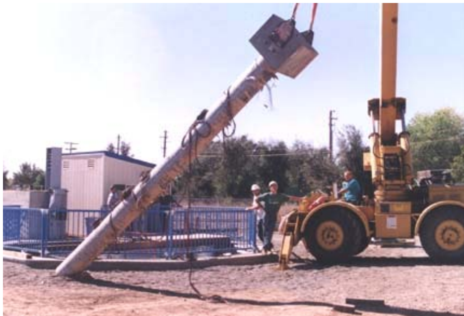
Figure 4-11 Precast Concrete Pile [39]
