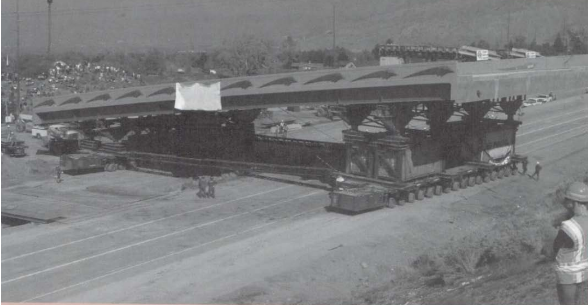
Figure 4-60 Transportation of Bridge Segment Using Self Propelled Modular Transporter [51]
