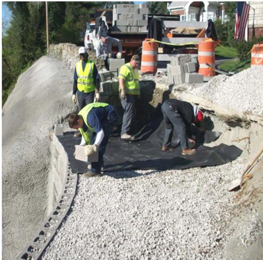
Figure 4-6 Installation of Geosynthetically Confined Soil Wall [19]
