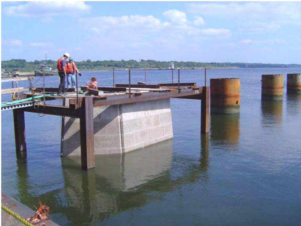
Figure 4-15 Bridge Pier Box (Photo courtesy of Cardi Corporation) [14]
