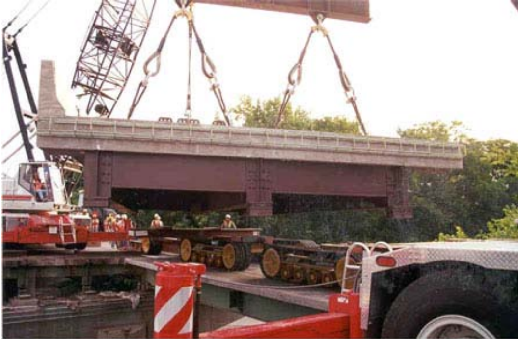
Figure 4-44 Unloading Pretopped Girder System for I-95 Bridge in Virginia [56]
