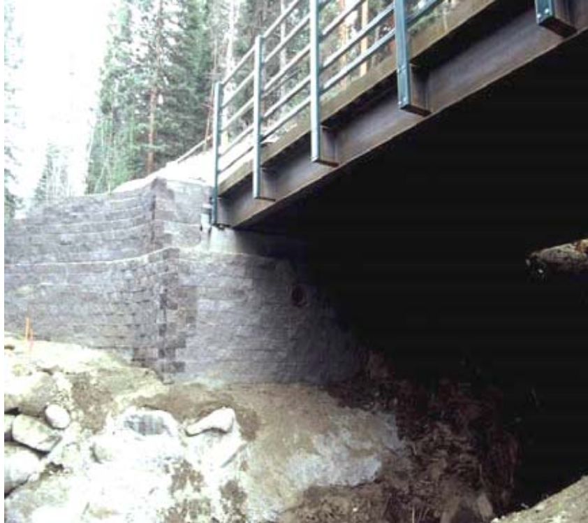
Figure 4-7 Geosynthetically Confined Soil Bridge Abutment [18]
