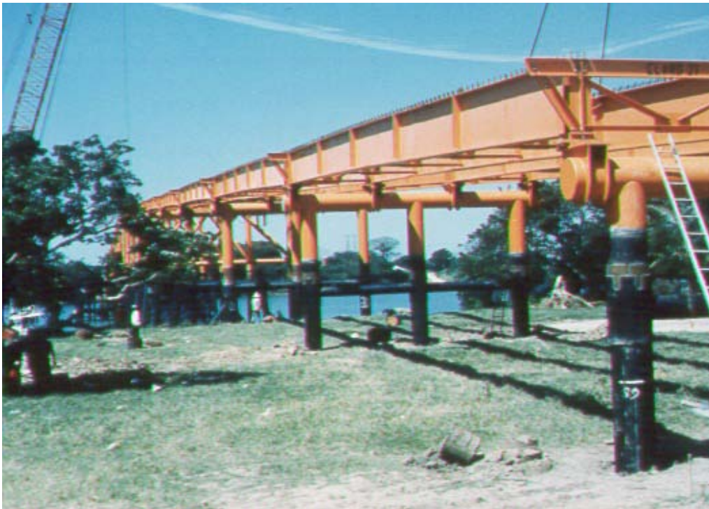
Figure 4-14 Modular Steel Piers [40]
