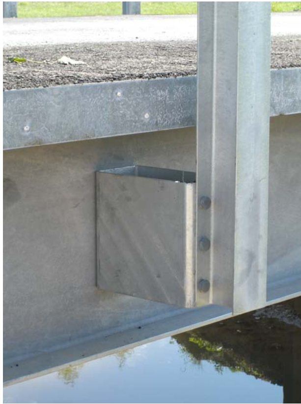
Figure 4-54 Steel Beam Rail Connection (U.S. Bridge Tour)
