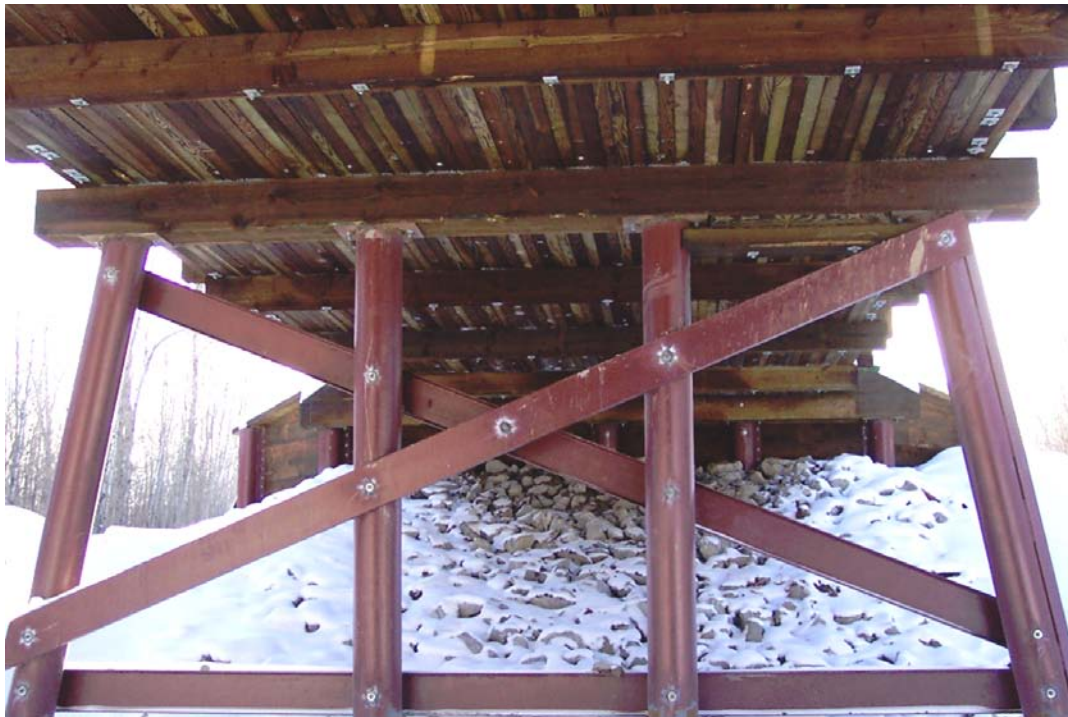
Figure 4-13 Driven Steel Piles for Piers/Abutments [12]
