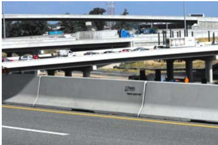
Figure 4-55 Precast Concrete Bridge Barrier [49]
