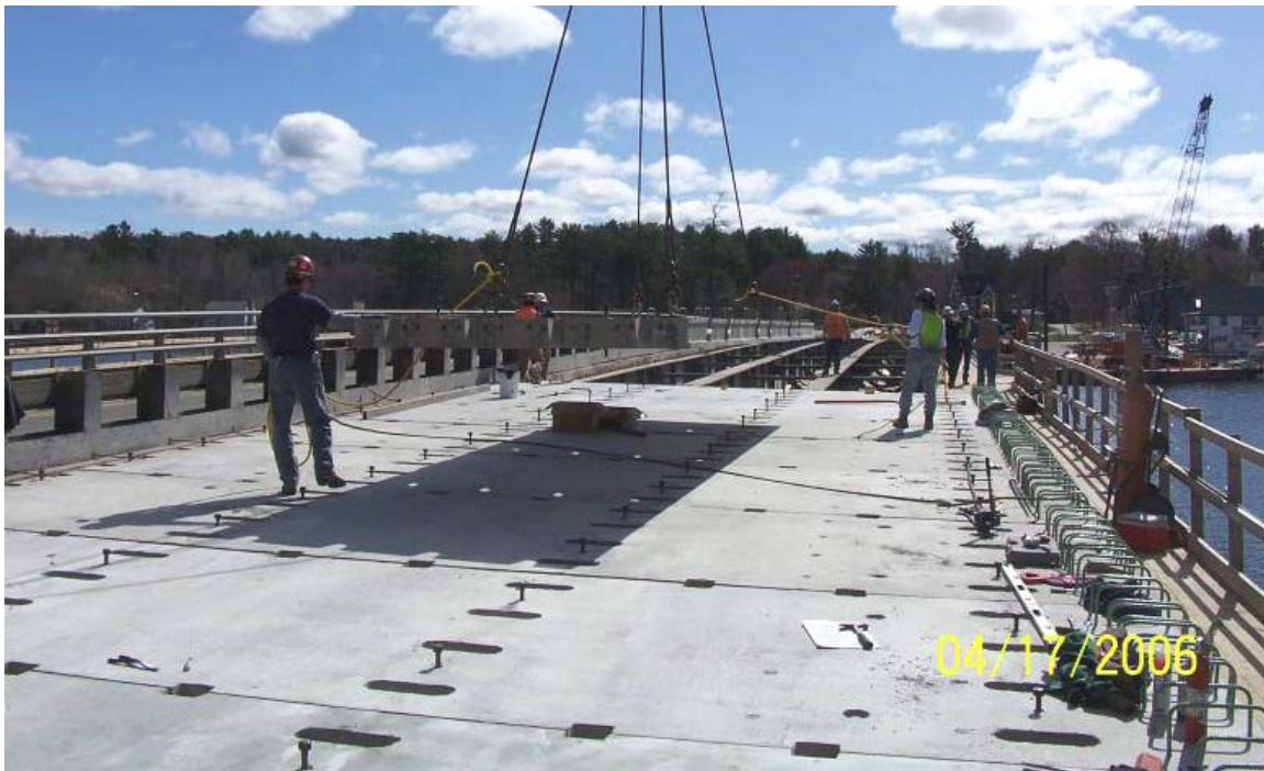
Figure 4-29 Full Depth Precast Deck Panels [14]
