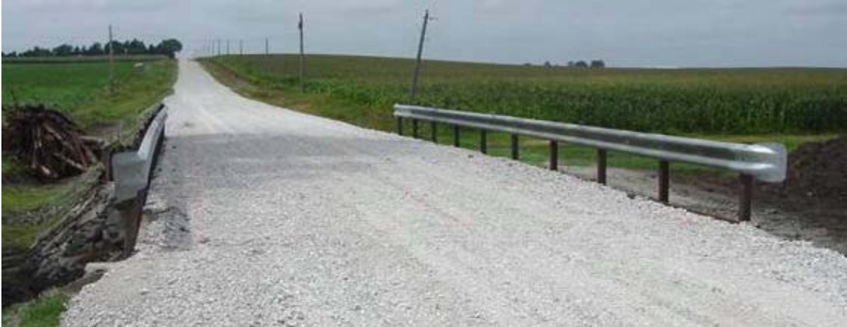
Figure 4-50 End View of Railroad Flatcar Bridge [57]
