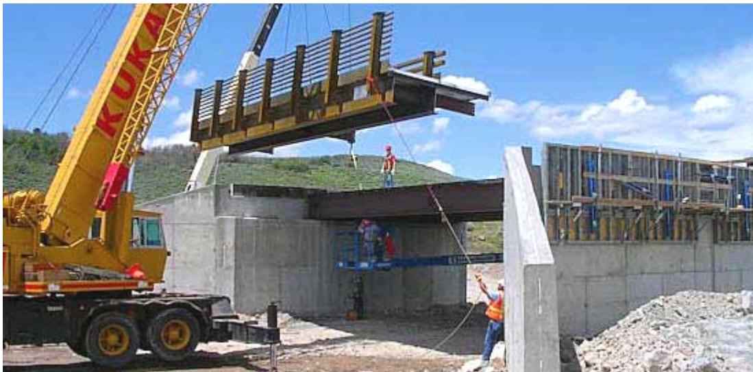
Figure 4-43 Assembly of Pretopped Girder Section Built by Big R Bridge [7]
