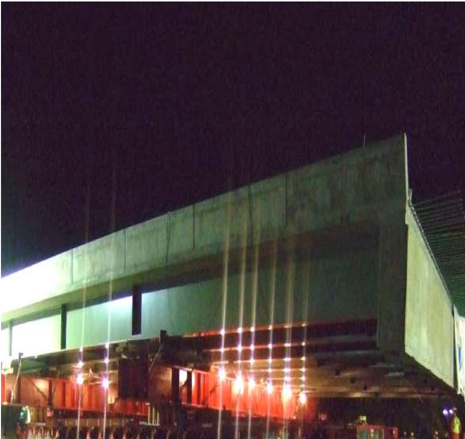
Figure 4-59 Self Propelled Modular Transporter [38]
