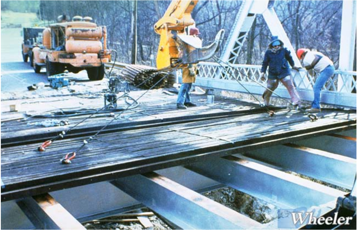
Figure 4-34 Installation of Transverse Timber Deck onto Steel Stringers [52]
