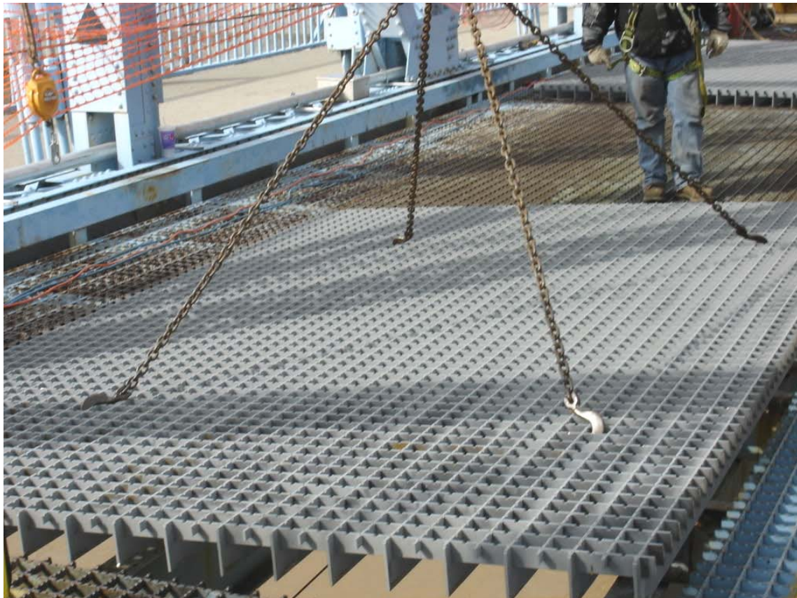
Figure 4-30 Open Grid Decking Being Placed [37]
