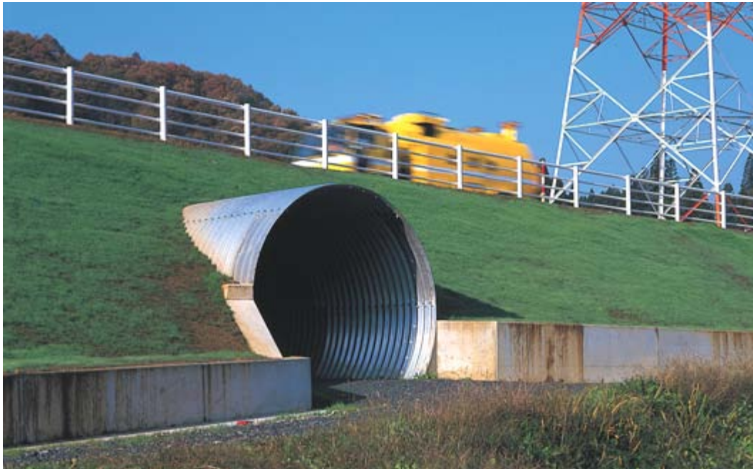
Figure 4-19 Corrugated Steel Pipe for Bridge Superstructure [15]
