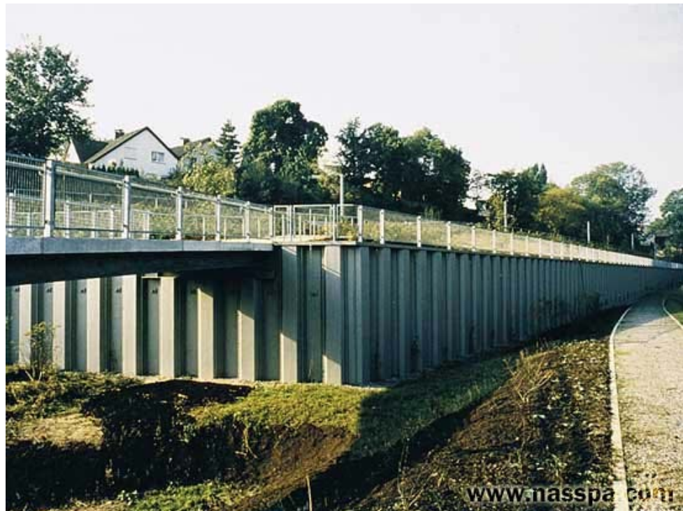
Figure 4-17 Steel Sheet Pile Wall Abutment [35]
