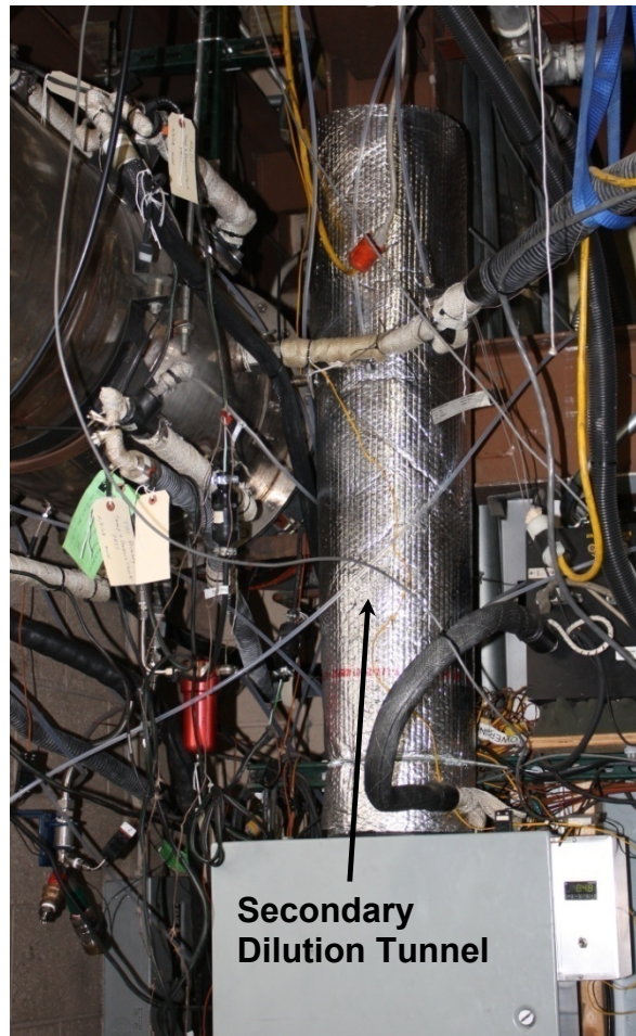
Figure 3.8 : Secondary Dilution Tunnel for PM Sampling.
