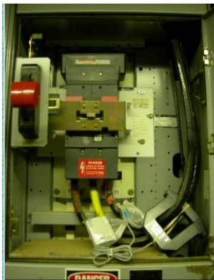
Figure 3.11: Data Logger and Current Transducer Setup
