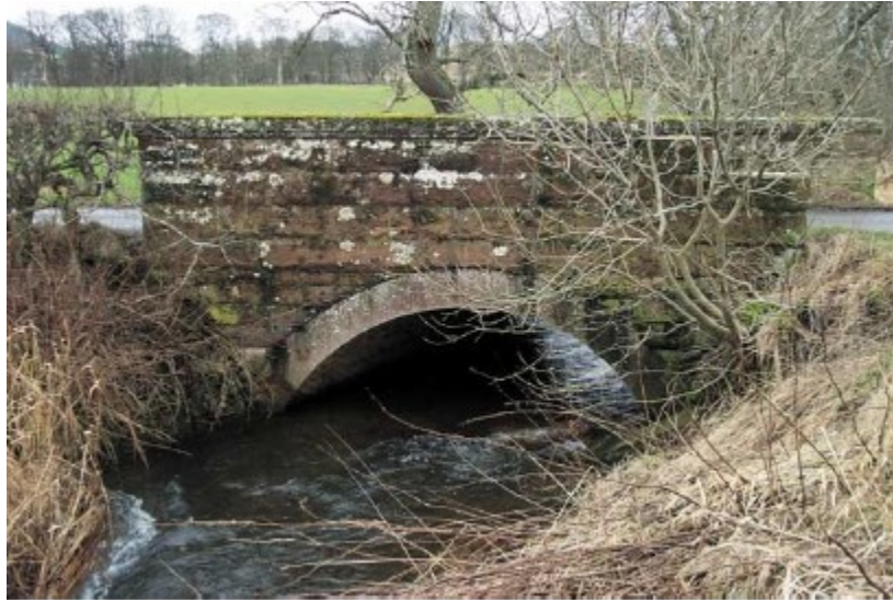
Figure 2.12: East side of the Kilbucho bridge (Clark et al. 2003).
