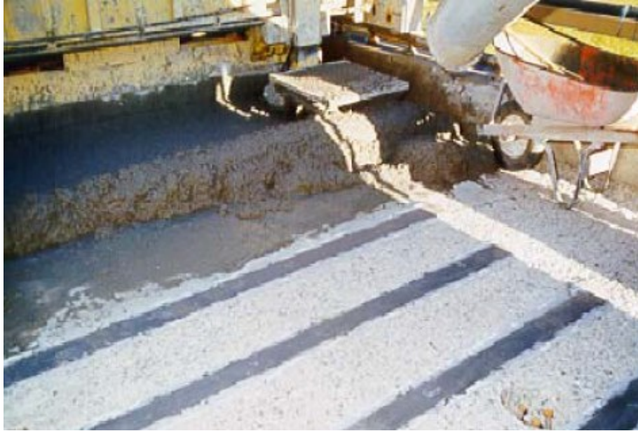
Figure 2.34: CFRP strips applied to existing deck (Hutchinson et al. 2003).
