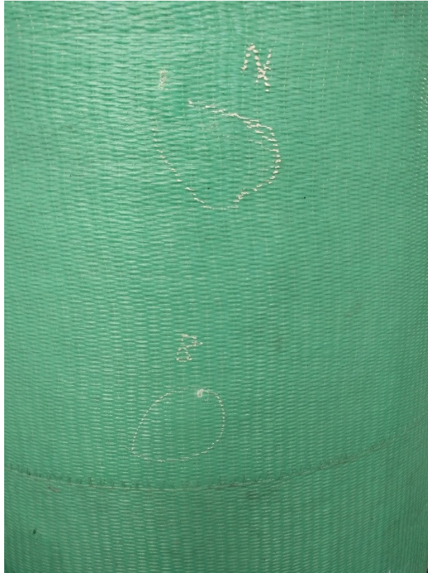
Figure 4.15: Regions 7 and 8 of center column in pier 3.
