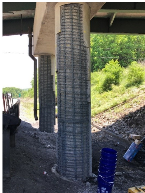
Figure 3.4: Pier 3 prior to patchwork.
