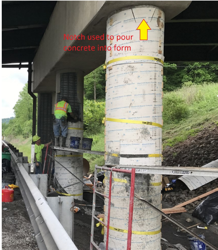
Figure 3.8: Concrete formwork
