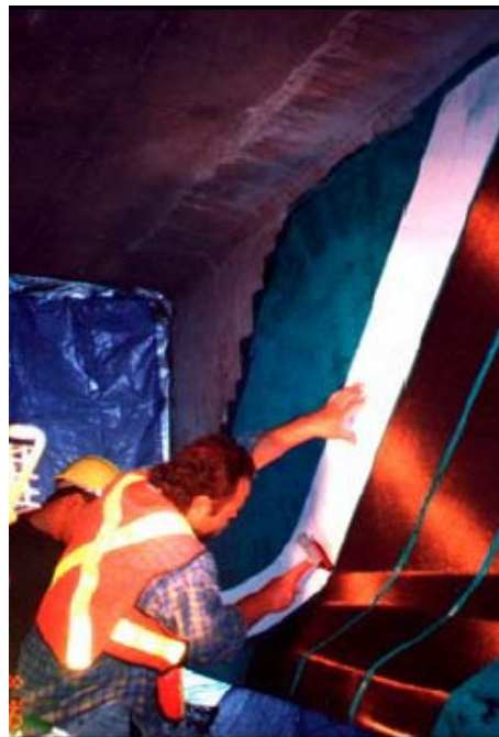
Figure 2.36: Application of the CFRP sheets (Hutchinson et al. 2003).
