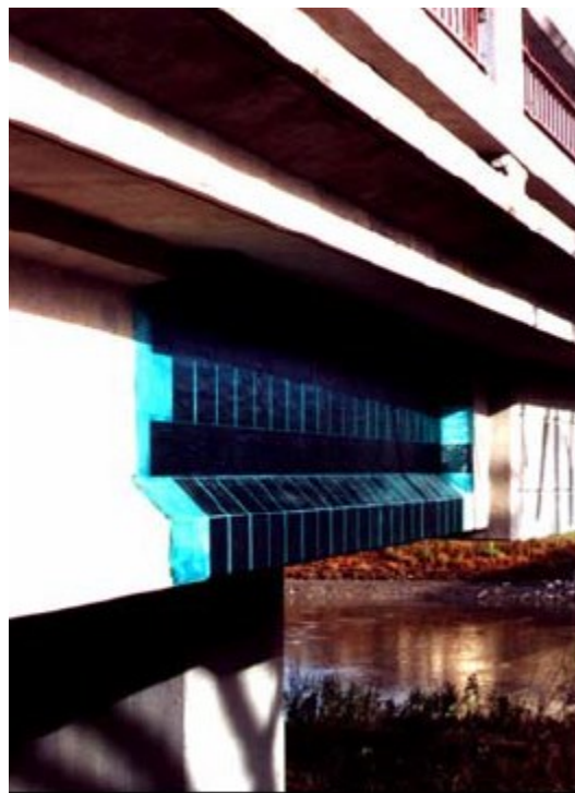
Figure 2.37: CFRP strips installed on the Maryland Bridge (Hutchinson et al. 2003).
