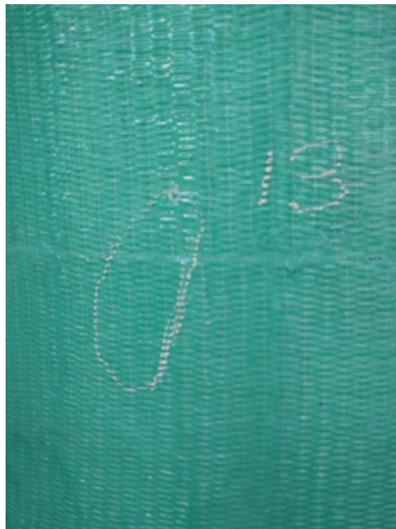
Figure 4.11: Area 13 on the center column of pier 3.
