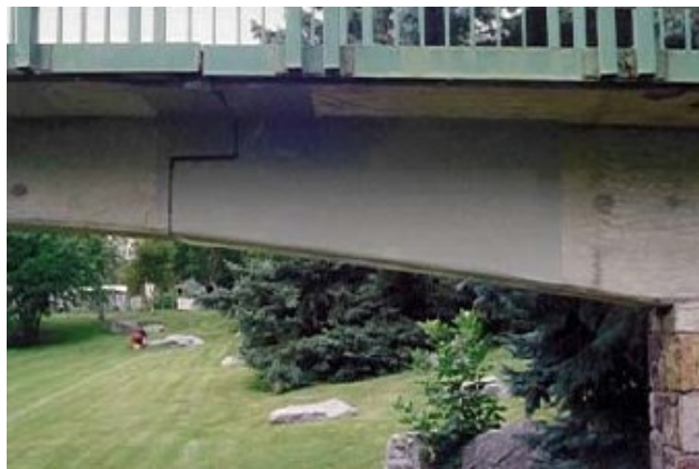
Figure 2.40: Jaques Lodge Bridge after corbel repairs (Hutchinson et al. 2003).
