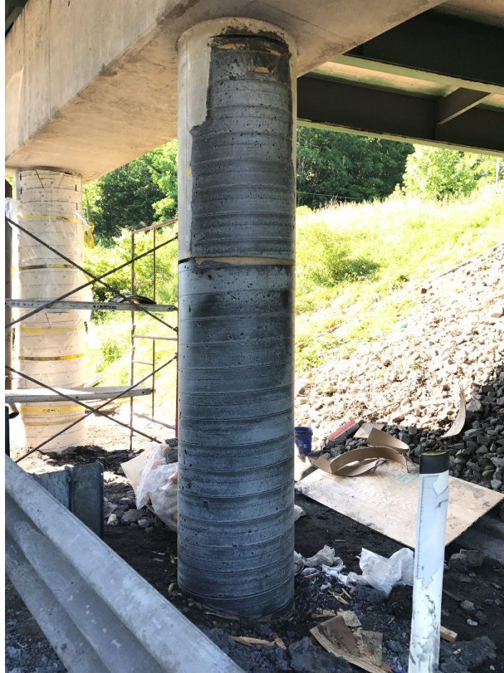
Figure 3.9: Concrete patchwork.
