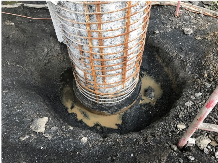
Figure 3.6: Excavation for patchwork.
