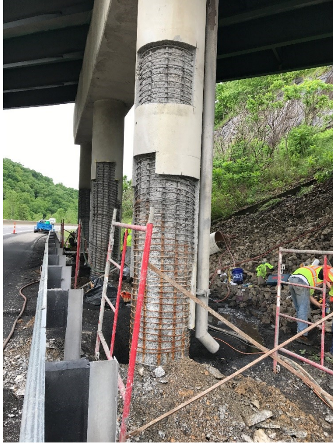
Figure 3.5: Pier 1 prior to patchwork.
