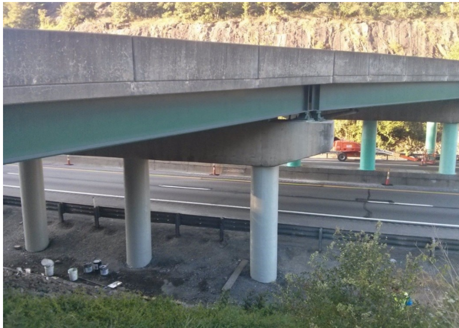
Figure 3.10: Completed Pier Set.
