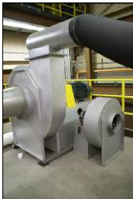
Figure 18 - Variable Speed Blower
