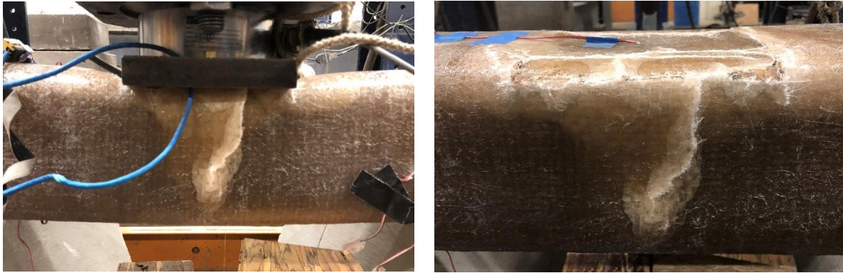
(a) (b) Figure 7-48. Failure on CB beams: (a) web crushing, (b) flange-web junction cracking
