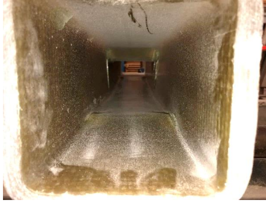
Figure 7-65. Stiffer bottom flange arresting bearing failure over the support on HFB beam
