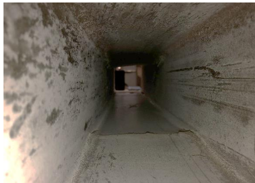
Figure 7-69. Transverse shear failure over supports on HAB beam
