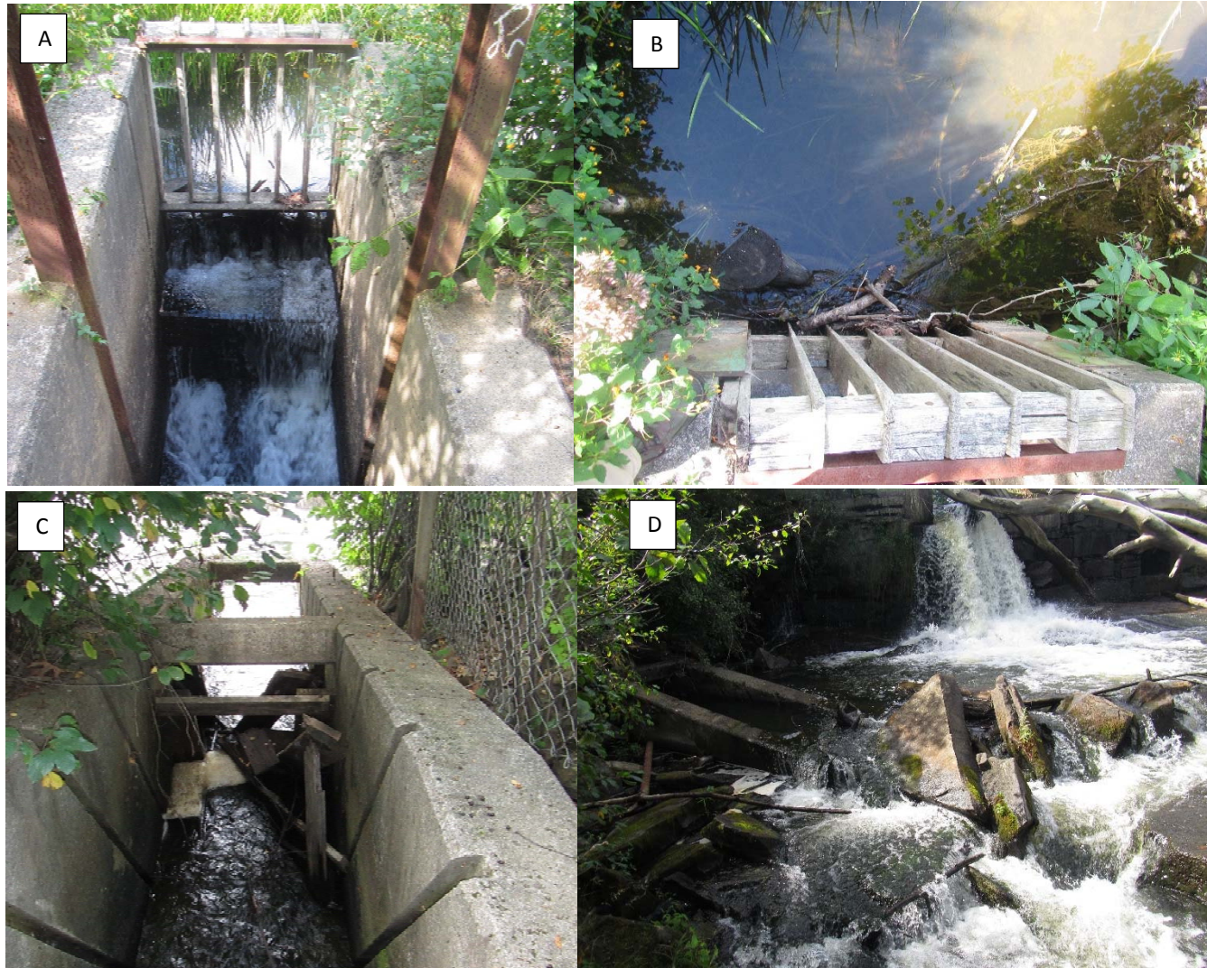
Figure 18: Selection of photos of East Elm Street Dam Fishway. (A) View is upstream at fishway exit into impoundment; (B) view of trashrack blocked by debris; (C) view is downstream at second baffle section blocked by broken baffles and debris; (D) entrance to fishway blocked by large wood and rubble.
