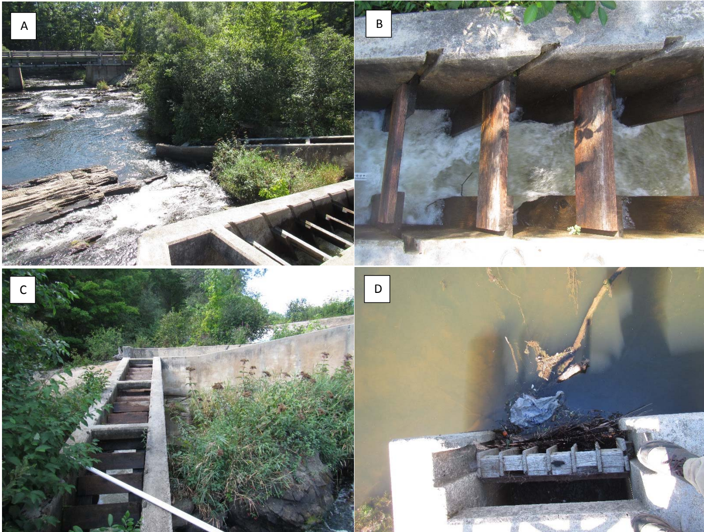
Figure 17: Selection of photos of Bridge Street Dam Fishway. (A) View is downstream at fishway entrance on river right. (B) View at a sample baffle section showing turbulent streaming flow. Flow is from right to left. (C) View is upstream towards first baffle section, with second baffle section extending towards the right. (D) Exit of fishway into impoundment showing trash and debris blockage.
