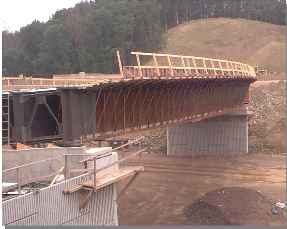
Figure 1-5. Deck forming brackets on exterior girders
