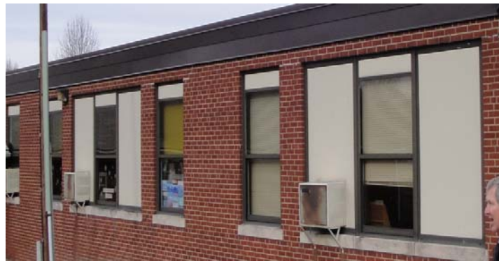
Figure 3.2 Checking the Belmont Elementary School Windows during Audit
