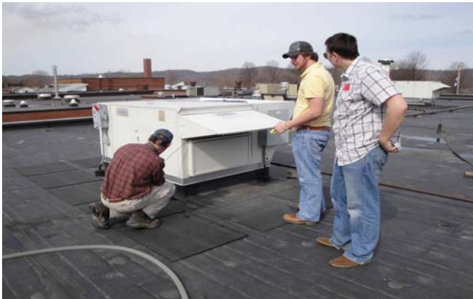
Figure 1.3 Measuring the Intake Air flow through the Dampers
