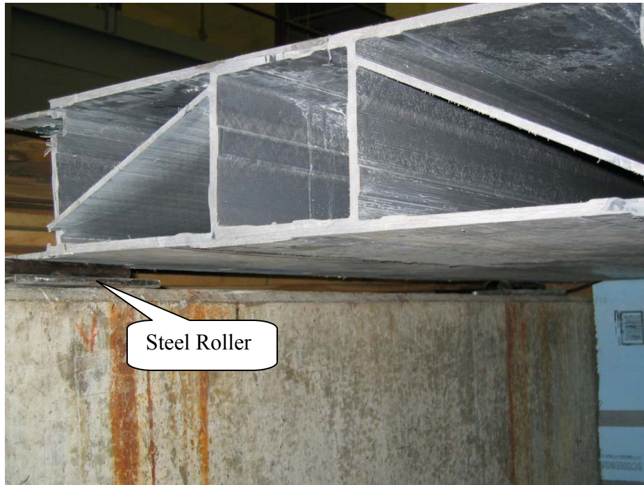
Figure 4.7: Steel Roller at the Corner of the FRP Deck.
