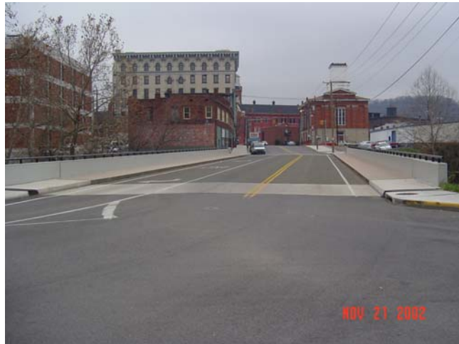
Figure 1.5: Market Street Bridge – Open to Traffic.
