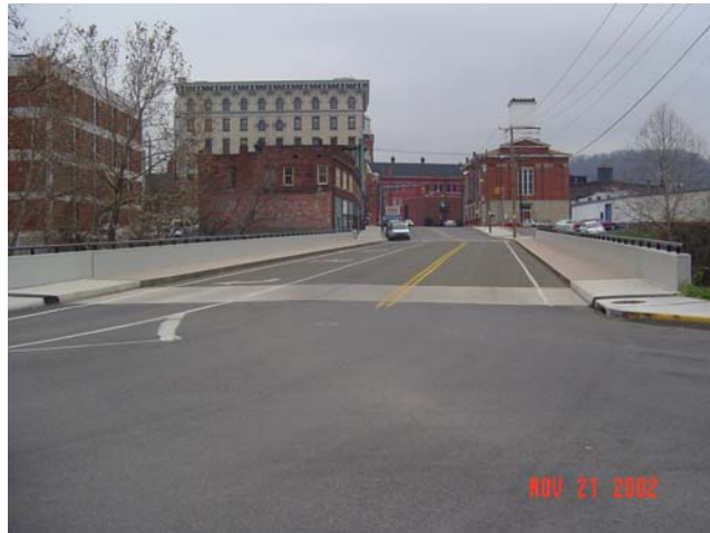
Figure 6.4: View After Applying Polymer Concrete (Market Street Bridge).
