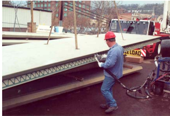
Figure 1.4: Applying Pliogrip Adhesive to a FRP Deck Module.
