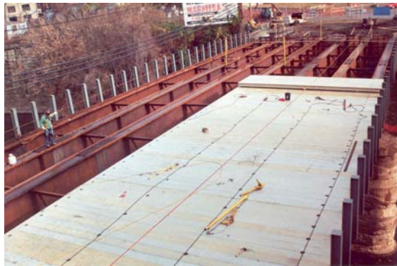
Figure 1.1: Installing FRP Deck on steel stringer.
