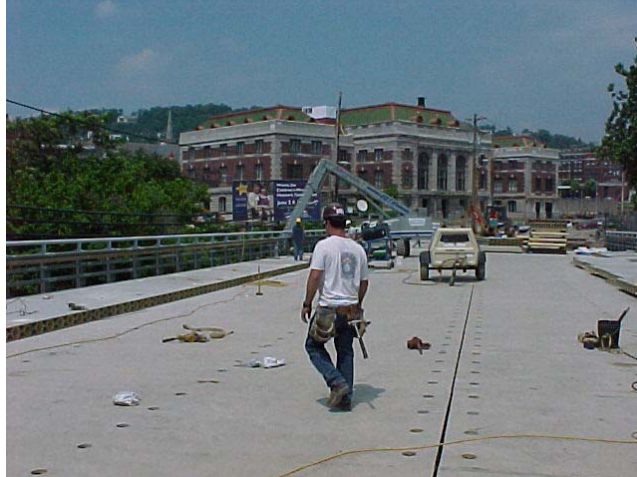
Figure 6.3: View Before Applying Polymer Concrete (Market Street bridge).
