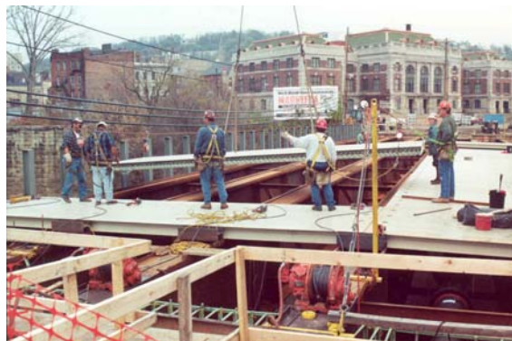
Figure 1.2: Using Nylon Strap to Lift FRP Deck.
